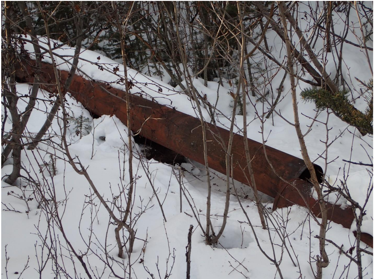
Steel Drainage Culvert – photo taken March 2016
