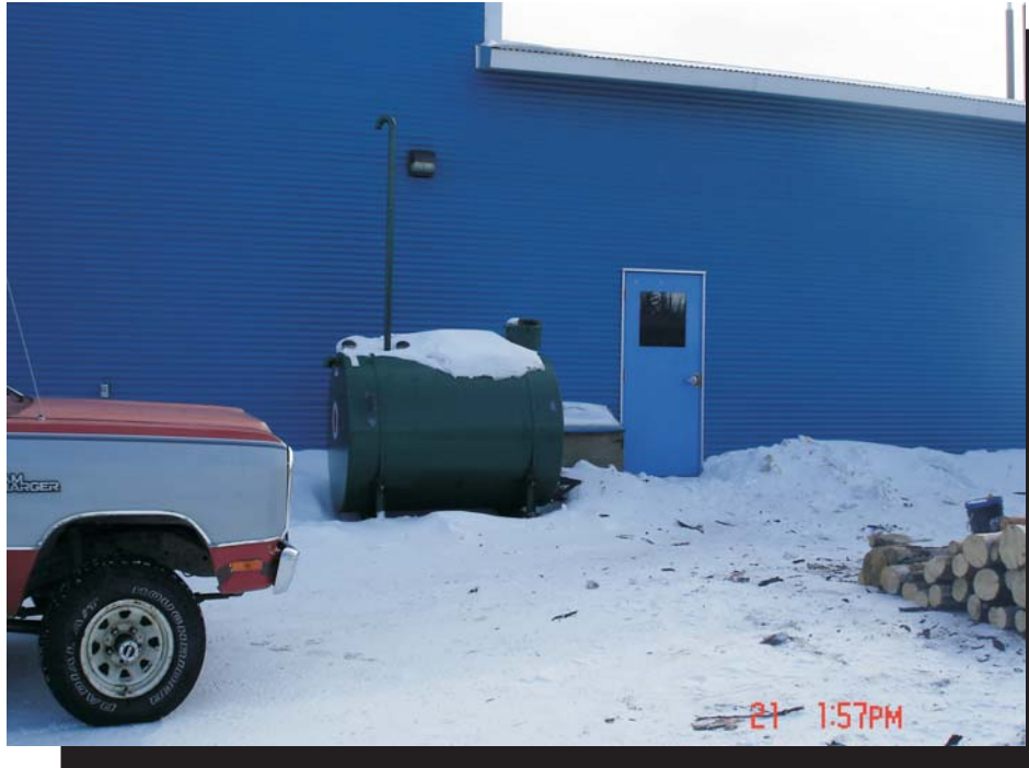
Photograph 3 AST adjacent to Water Truck Garage and KFN-F (March 21, 2007)
