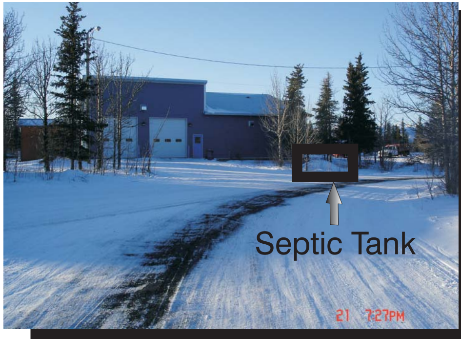
Photograph 1 Water Truck Garage; Septic tank located in front of Garage (March 21, 2007)
