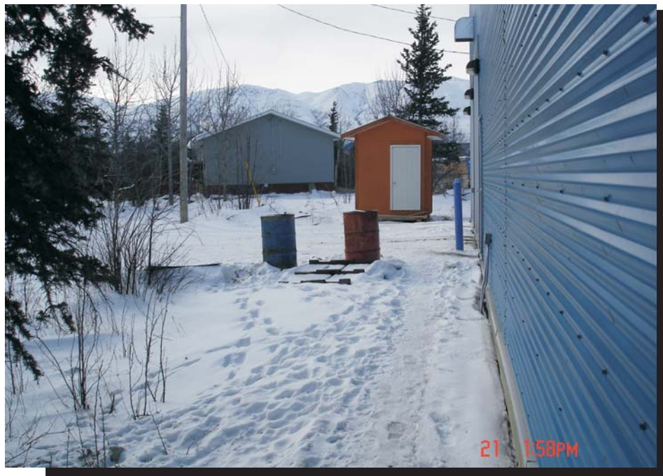
Photograph 4 200 L fuel drums adjacent to the west die of the Water Truck Garage; no secondary containment. (March 21, 2007)
