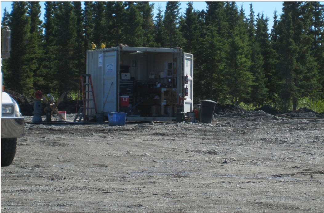
Photo 2: KFN-K and KFN-L during final pumping testing. August 23, 2012
