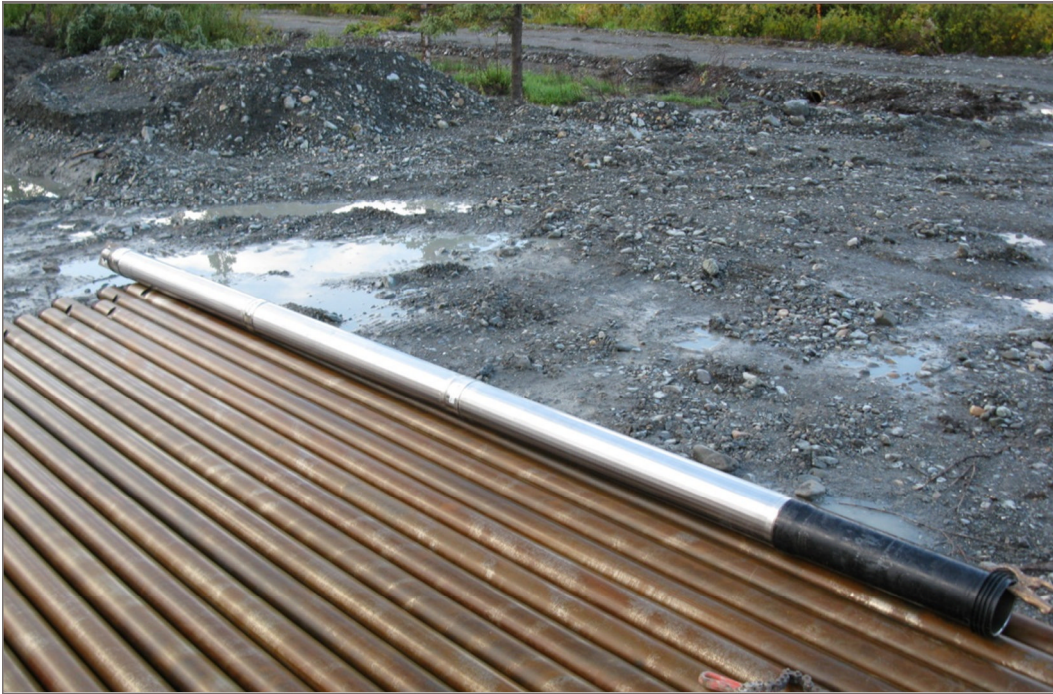
Photo 3: KFN-L 10-slot well screen, riser and K-packer prior to installation. August 19, 2012
