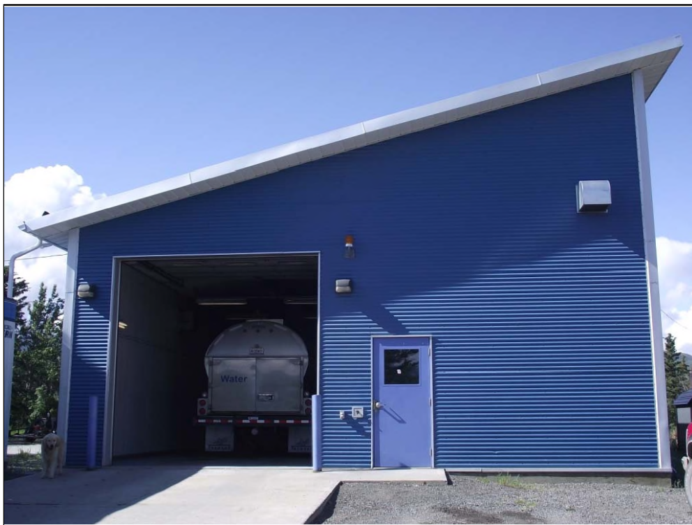
Photo 1: Water Truck Garage (north end). July 2011. Note: A larger truck as desired by KFN would not fit within current geometry.
