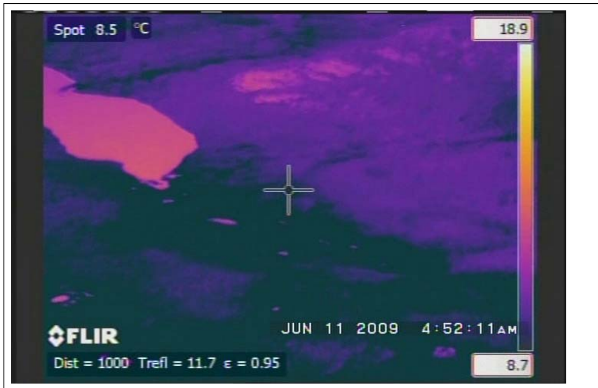
Thermogram # 14. Jarvis Area Water Samples Location (Figure 3). Video reference 4:52:11 AM.
