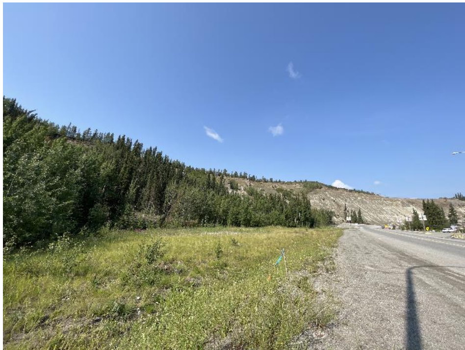
Photograph 4. Erosion area, showing transition from moderate (left foreground) to high (right background) constraint with a transition from stabilizing vegetation to a lack of vegetation, respectively.
