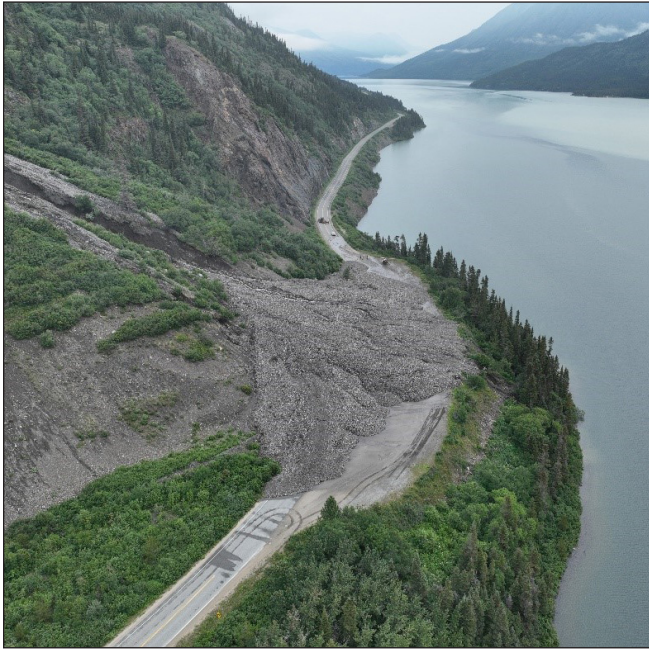
Figure 9. Photo (view to north) of landslide on the South Klondike Highway by Tutshi Lake.
