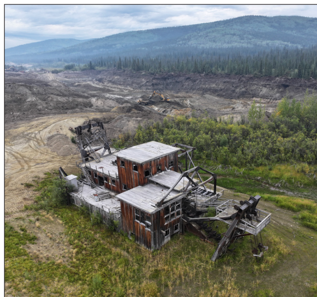
Figure 9. YCGC Dredge No. 8 on the mid reach of Sulphur Creek. Schmidt Mining's active cut is visible in the background.
