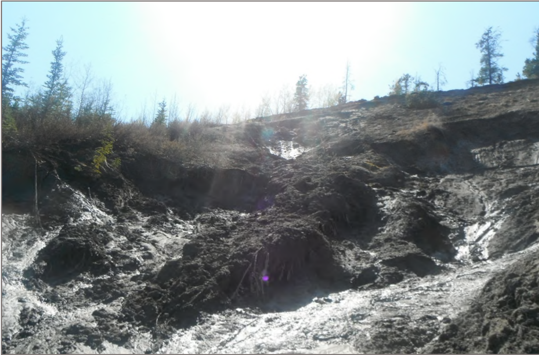
Photo 1: Three of the four back scarps at the site (May 15, 2014)
