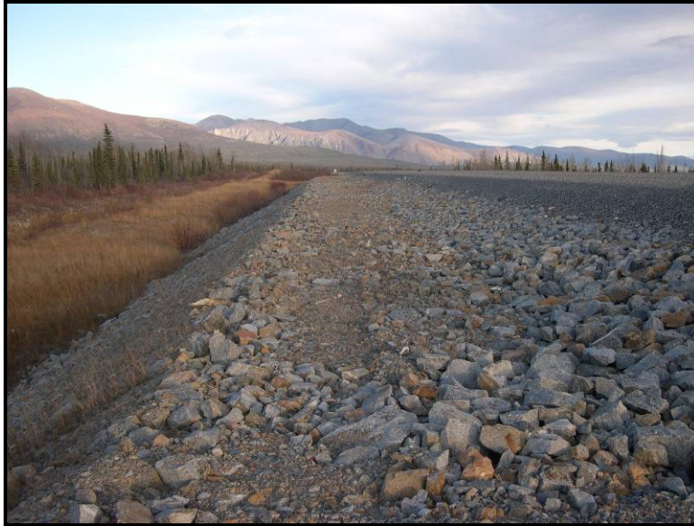
Figure 2-20: Rock Berm on Alaska Highway, Yukon, Canada (Photo by Guy Doré, Université Laval)
