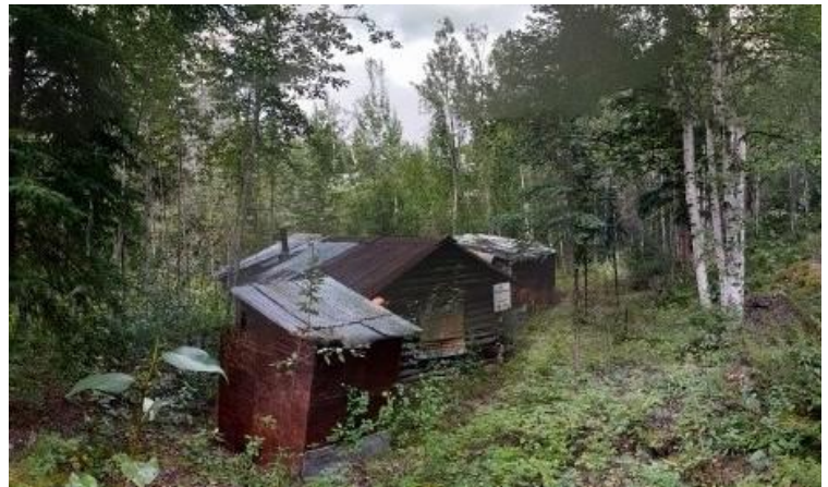
View of cabins in Area # 20 facing north-west.
