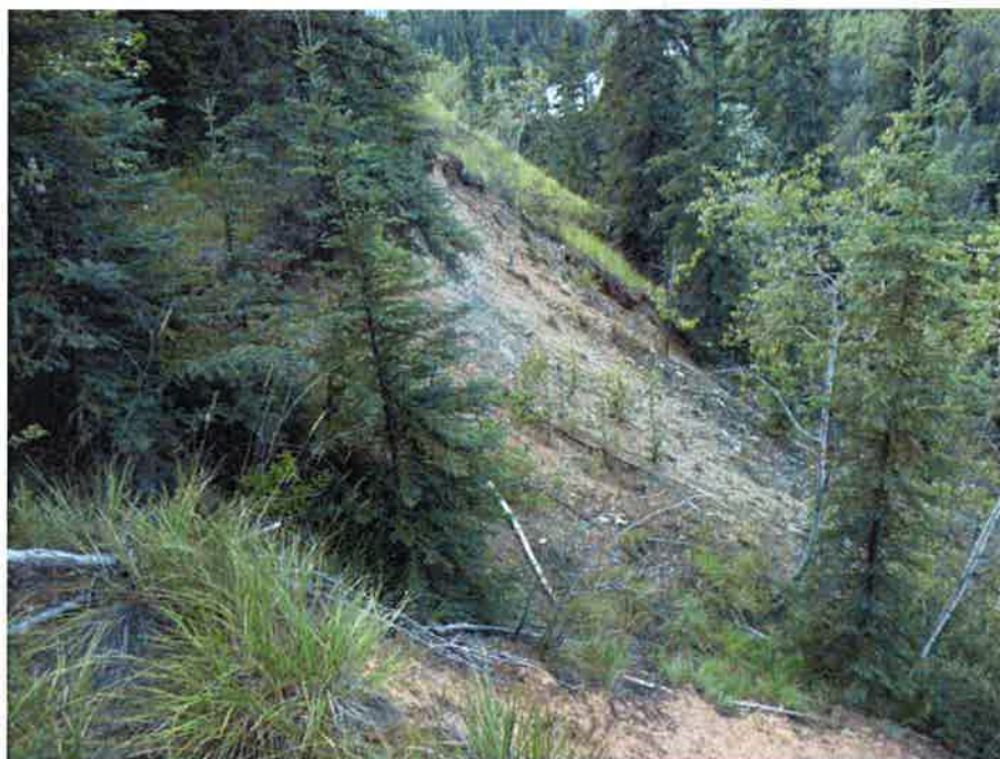
Photo 5: Minor erosion along escarpment. Most of the escarpment is vegetated as shown in distance.
