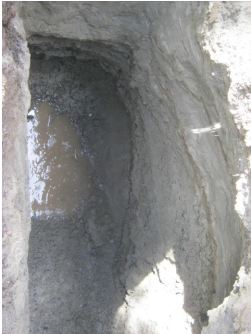
Figure 835-4809.4 Photo of Test Pit 835-4809, excavated July 2014.
