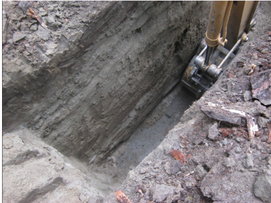
Figure 835-4812.5 Photo of Test Pit 835-4812, excavated July 2014.
