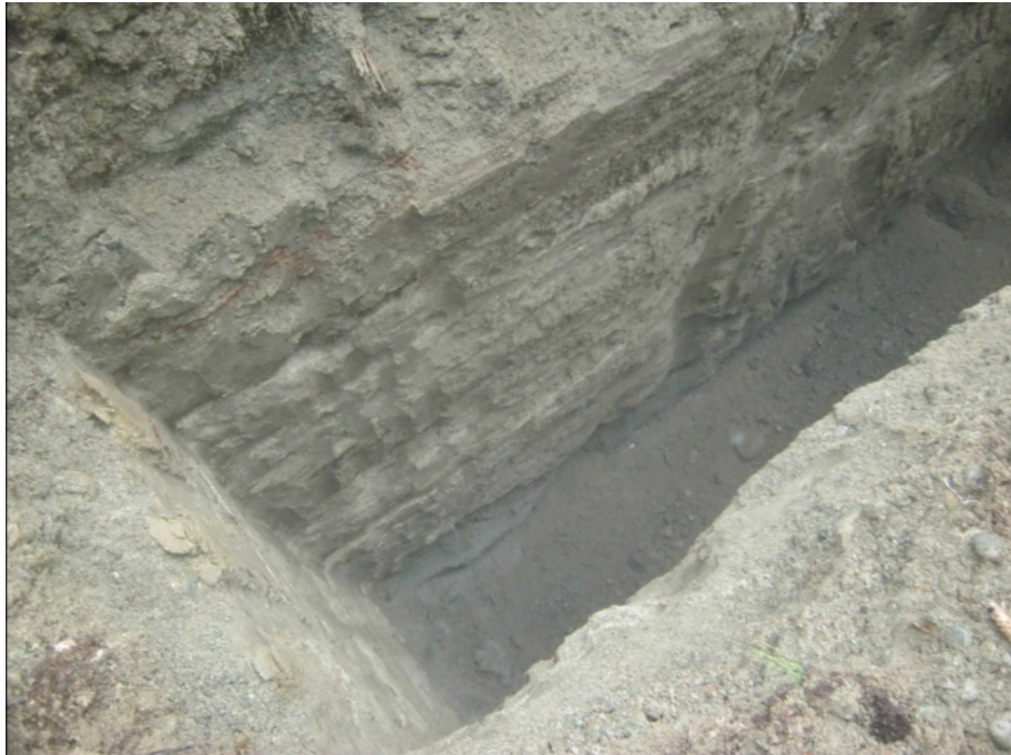
Figure 835-4814.4 Photo of Test Pit 835-4814, excavated July 2014.
