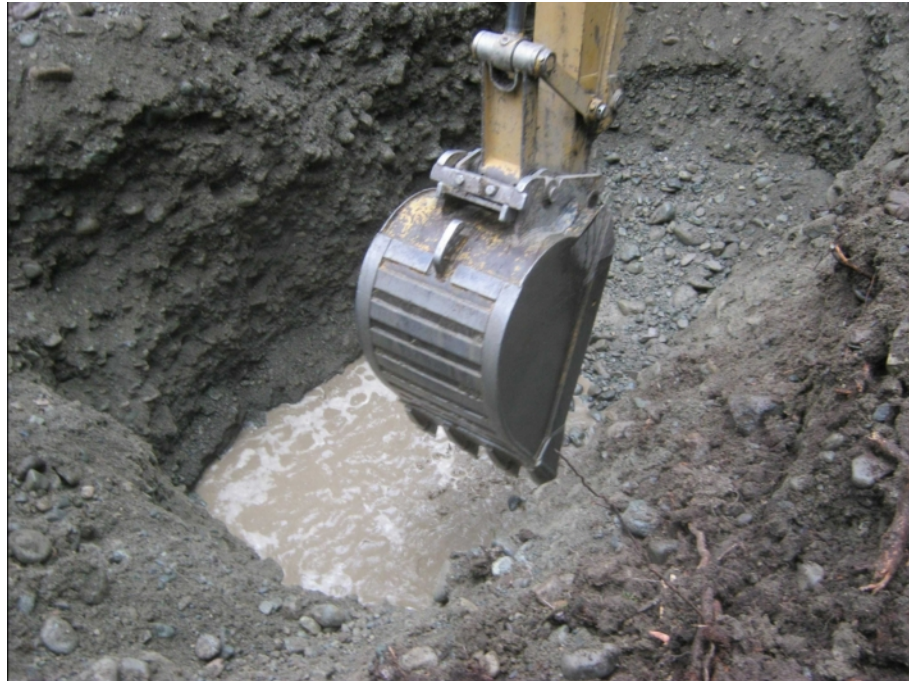
Figure 835-4806.1 Photo of sample piles from Test Pit 835-4806, excavated July 2014.
