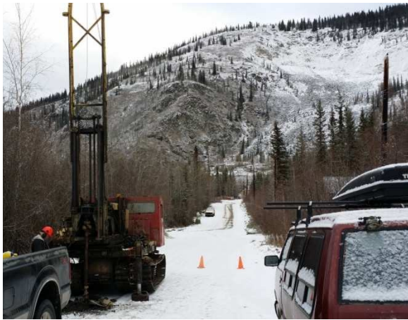
Photo # 1 (left) –BH 1-14 site conditions facing north from Edward Street.
