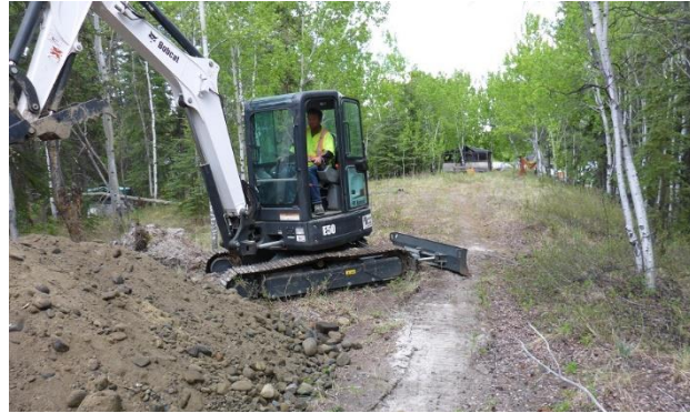
TP 1-18 – Facing North
