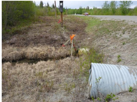
Culvert Inlets facing North
