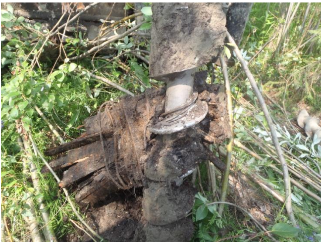
Photo # 2 – BH 1-14 Old wooden culvert at 1.0 meters
