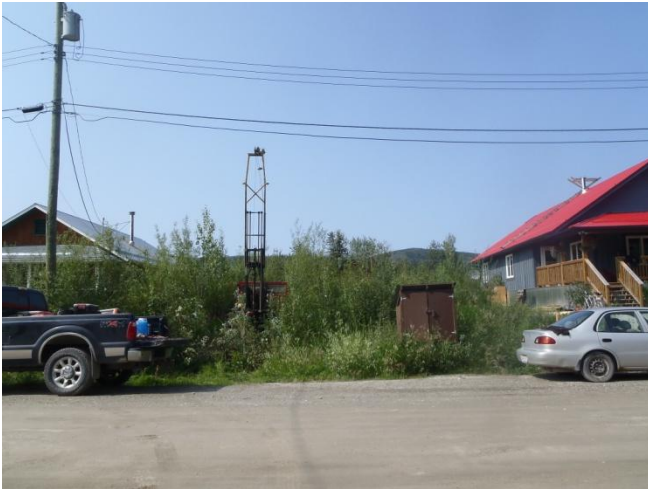
Photo # 1 – Site conditions during drilling operations facing west from Judge Street.
