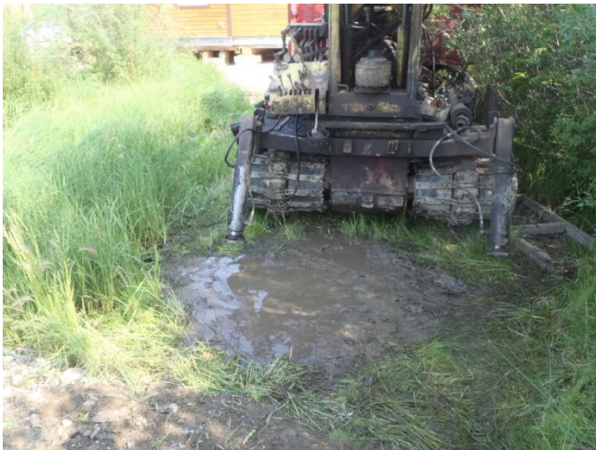
Photo # 3 – BH 1-14 – Site conditions upon completion of drilling operations.
