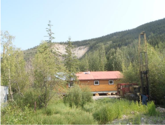
Photo # 1 – Site conditions during drilling operations facing north-east from Albert Street.
