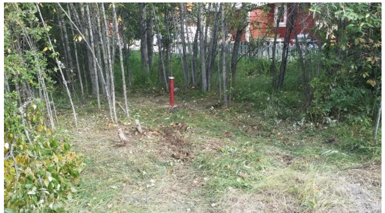
Photo # 4 (right) – Site conditions following well installation
