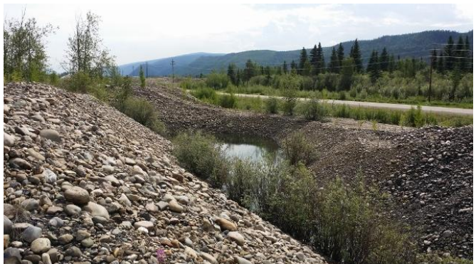
Photo # 5 - Conditions facing south-east towards Klondike Highway # 2
