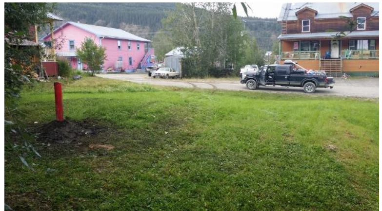
Photo # 4 (right) – Site conditions following well installation facing 7 th Avenue.
