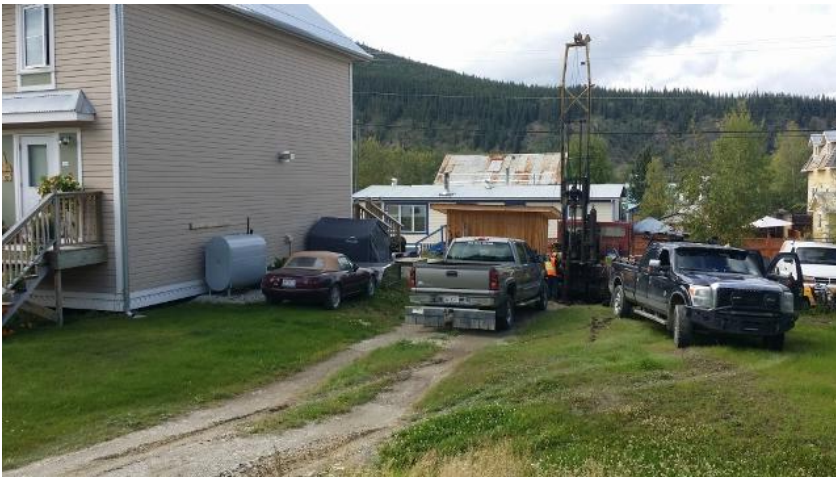
Photo # 1 (above) – Drilling BH 1-15 - As viewed from 7 th Ave.
