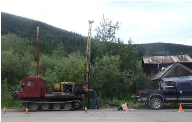
Photo # 1 – Site conditions during drilling operations facing west from Judge Street.
