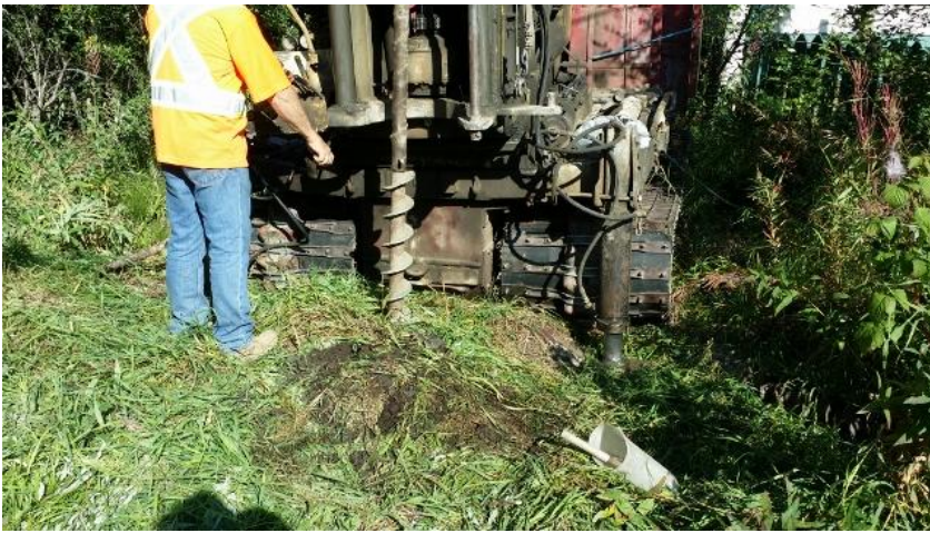
Photo # 1 (above) – Drilling BH 1-15
