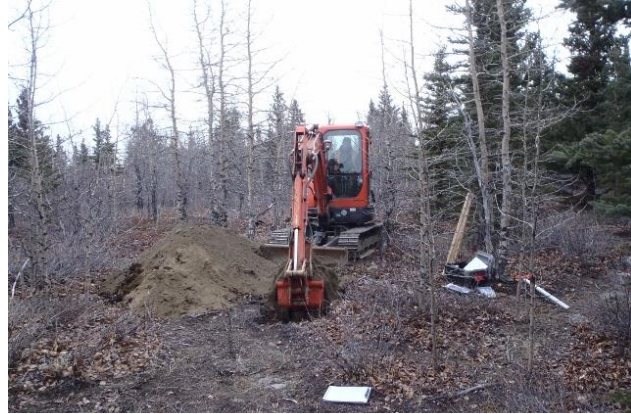
Excavation of TP 1-17
