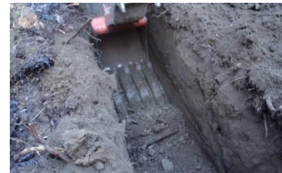
TP 5-17 Excavation conditions
