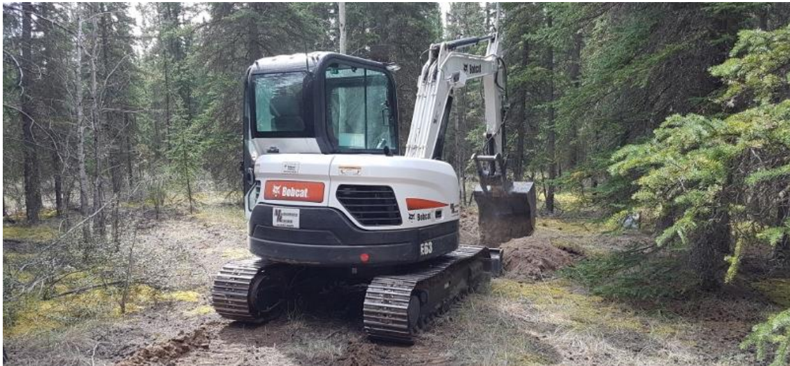
Backfilling test pit TP 6-19
