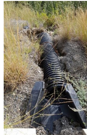
Discharge flume conditions
