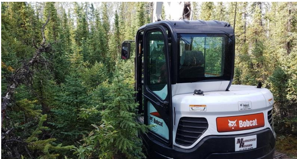
Site conditions traversing to test pit TP 2-19.
