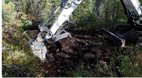
Backfilling test pit TP 1-19.
