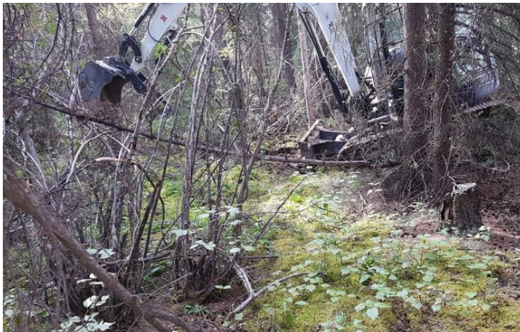
Site conditions at test pit TP 3-19.
