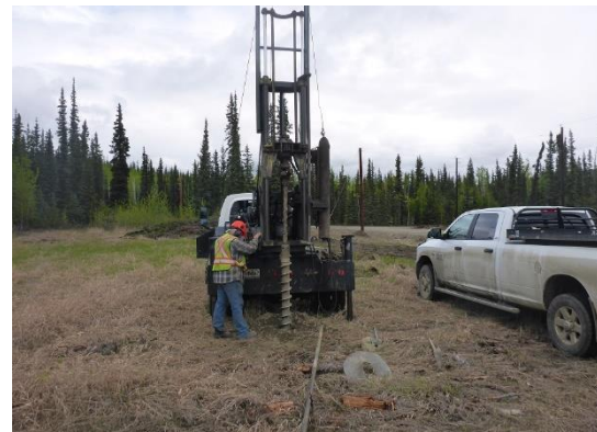
Auger drilling borehole BH 5-18
