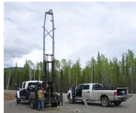
Drilling of borehole BH 6-18
