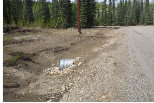
Outlet and ditch conditions at CSP 3.
