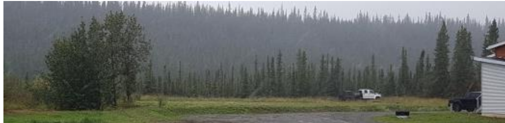
View of site from River Drive. Drilling borehole BH 2-19.
