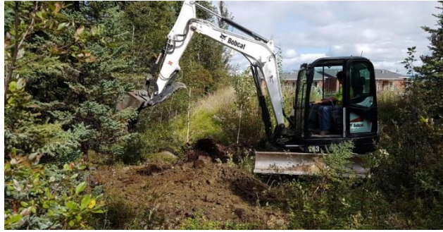
Backfilling test pit TP 3-19.
