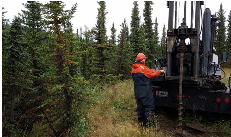
Drilling borehole BH 1-19.
