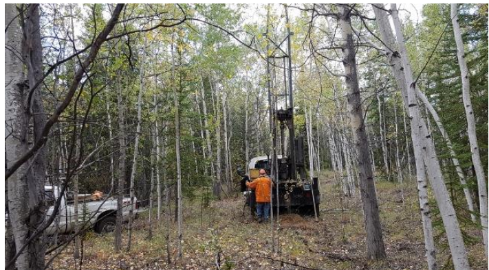
Borehole BH 3-19 – Field Conditions
