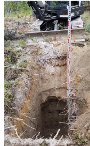
Test Pit TP 3-19
