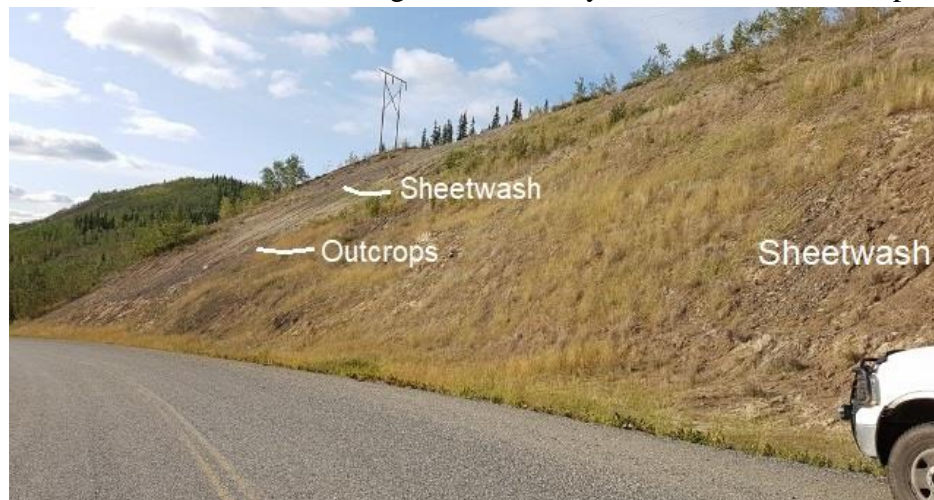
Western slope conditions facing northwest.
