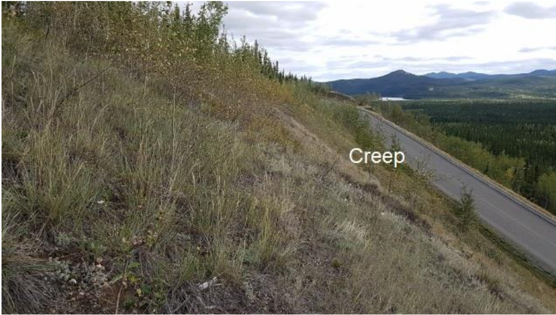
Central slope conditions facing southeast
