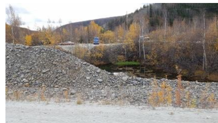
View of northwestern tailings pond from Rabbit Creek road.
