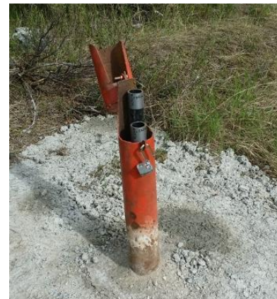
Borehole BH 5-17 Well and Casing
