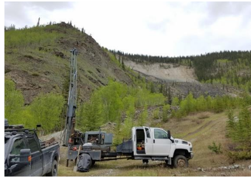
Borehole BH 5-17 facing east
