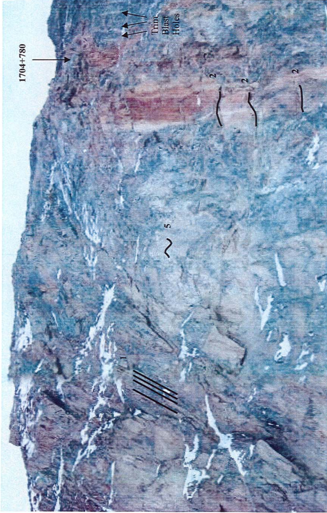
Photo 4: Structural Domain 2 (Quartzite) with selected joint sets highlighted. Note traces of small diameter trim blast holes spaced at approximately 0.8 m apart.
