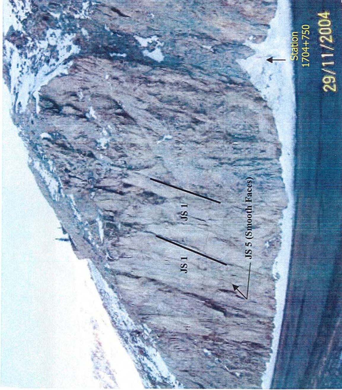
Photo 7: Locally pronounced joints of Joint Sets 1 and 5 in the quartzite in Design Sector 2.
