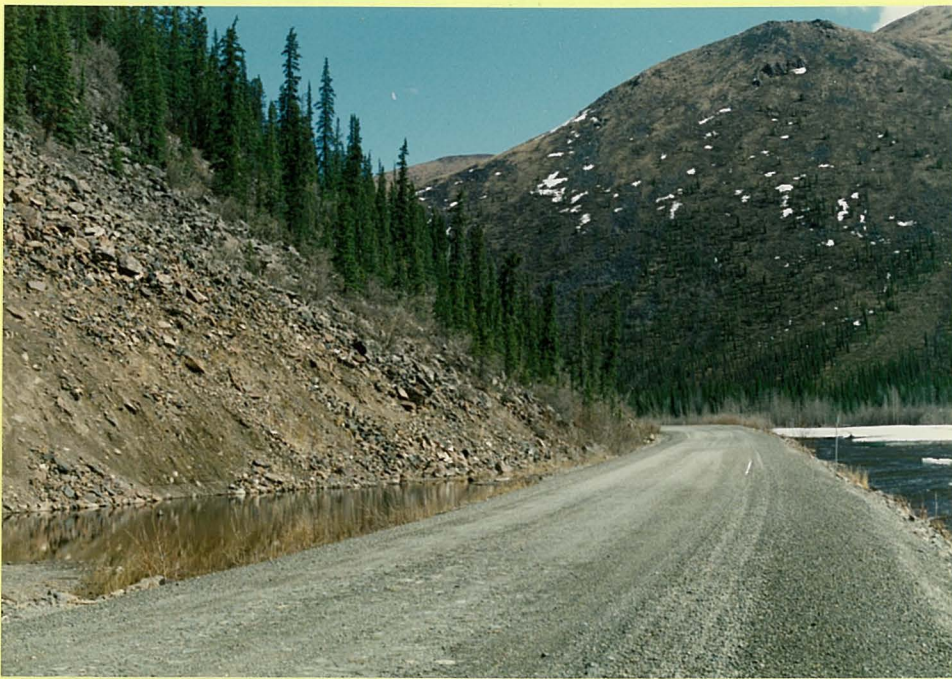
PHOTO 89-01-08 Dempster Highway Km 144 Looking north along highway. Talus slope to left, Blackstone River to right.
