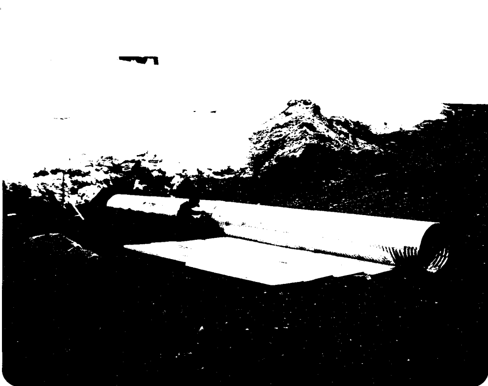
KM 46.9 INSTALLATION OF CULVERT EXTENSION AND PORTION OF 50 mm INSULATION
