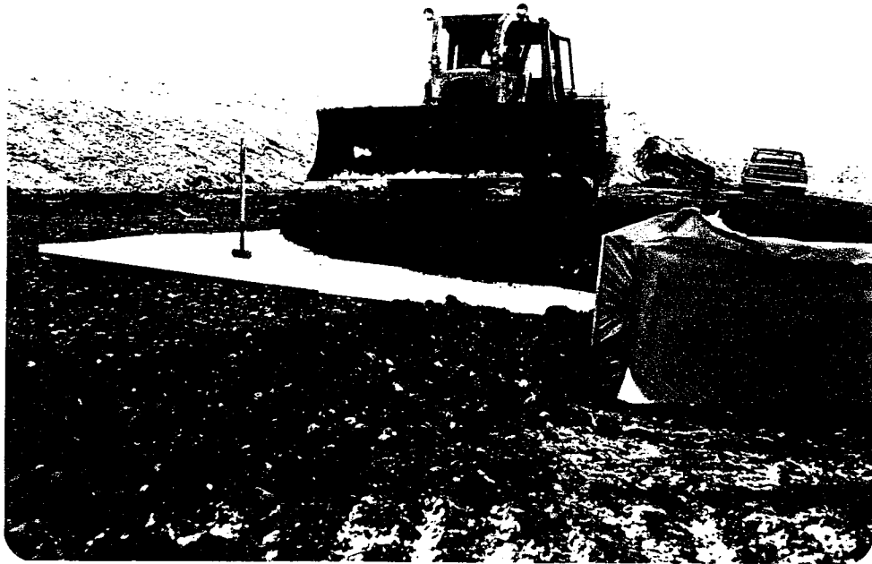
KM 50.9 PLACING LIFT OF FILL OVER 50 mm INSULATION
