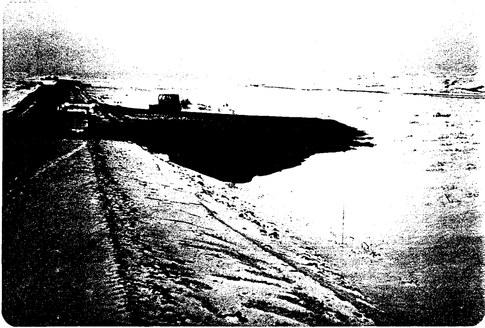
KM 50.9 PLACING FILL AT NORTH SIDE OF HIGHWAY - LOOKING WEST
