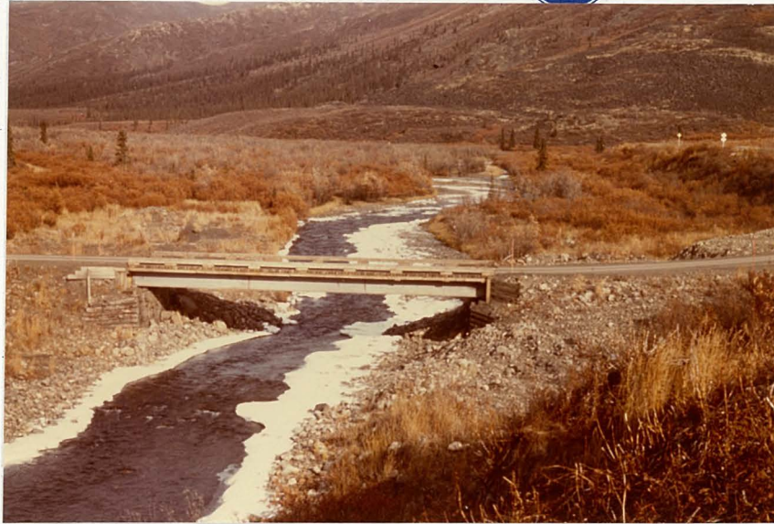
Photograph No. 9: The existing bridge where the road crosses the North Klondike River at approximately Mile 41.7. This view is looking upstream in a northerly direction. It is at approximately this point along the highway that the road passes out of the zone of thick spruce forest and into an area of scrub and alpine tundra.
