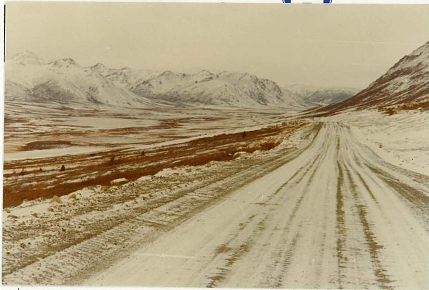
Photograph No. 13: Looking northerly from approximately Mile 50 near the "summit" which is the highest point between Mile 0 and Mile 78.
