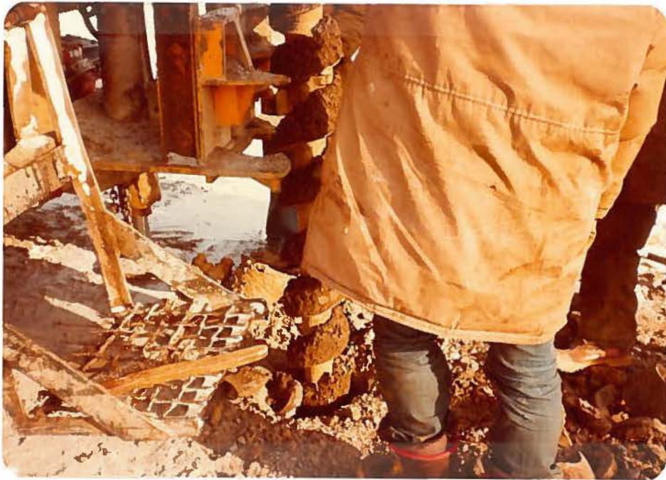
5. The D.P.W. drill crew taking a core sample at Station 1023+00.
