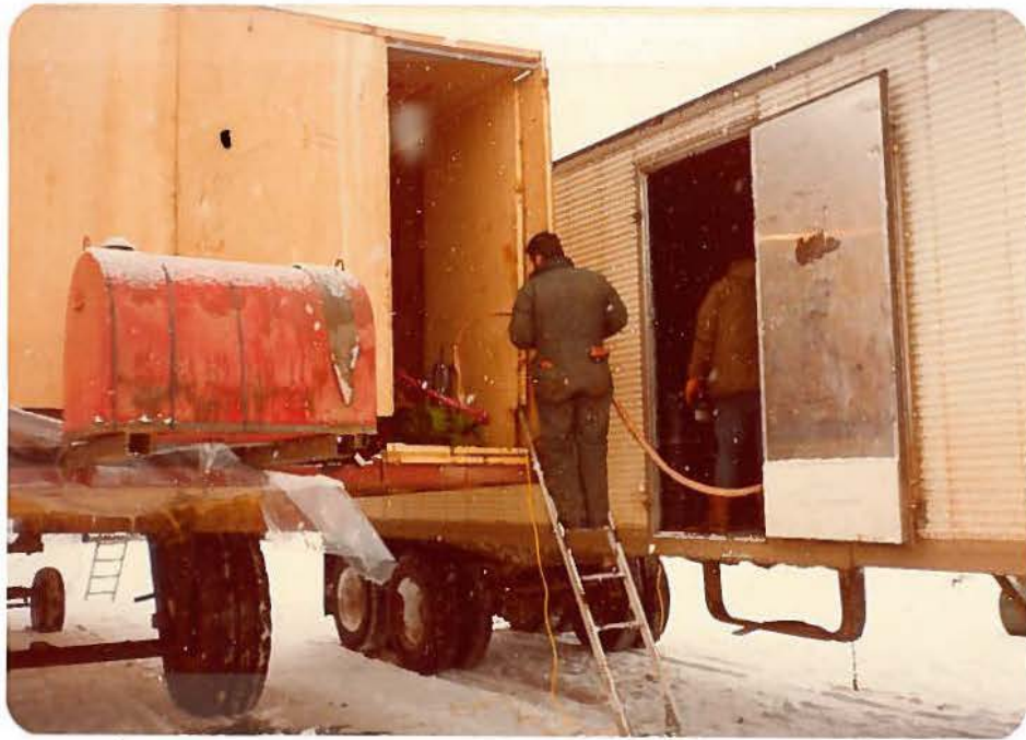
13. Pumping the foam producing liquids from 45 gallon drums to the machine. The liquids were not warm and so presented difficulty pumping.
