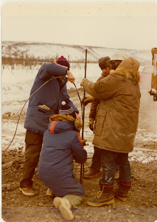
8. The installation of the monitoring system by NRC. The thermistor cables reach to a depth of about eleven (11) feet with thermistors at one to two foot intervals.
