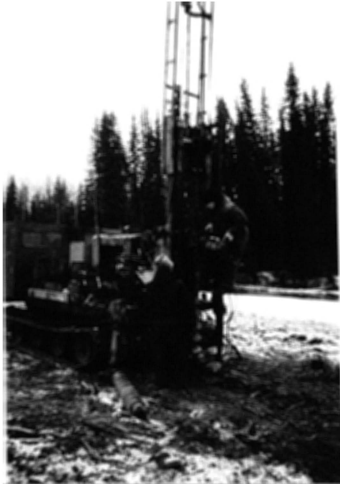
PHOTO # 3 – T.H. # 9A-98 Maintaining positive head during drilling operations
