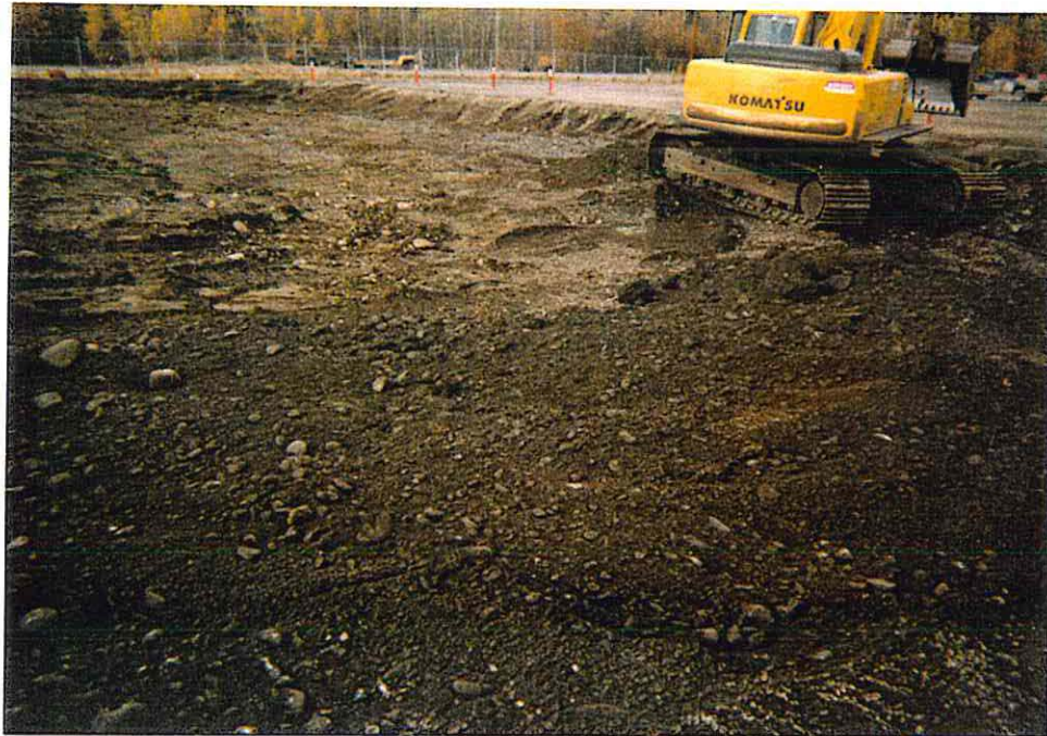
PHOTO # 14 – Repair Area 3-2 – Excavation Base
