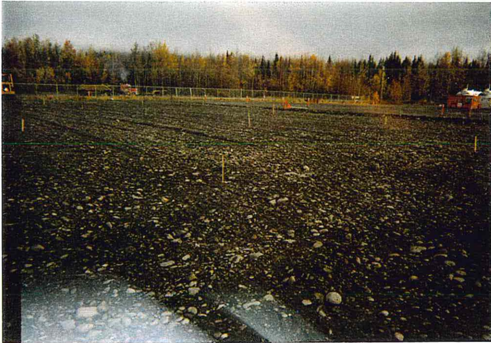
PHOTO # 16 – Repair Area 3-2 – Preliminary Grading near top of Granular E
