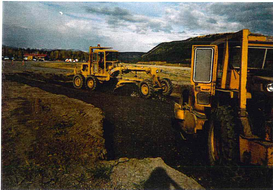
PHOTO # 6 – Repair Area 1 – Granular E Backfill Operations
