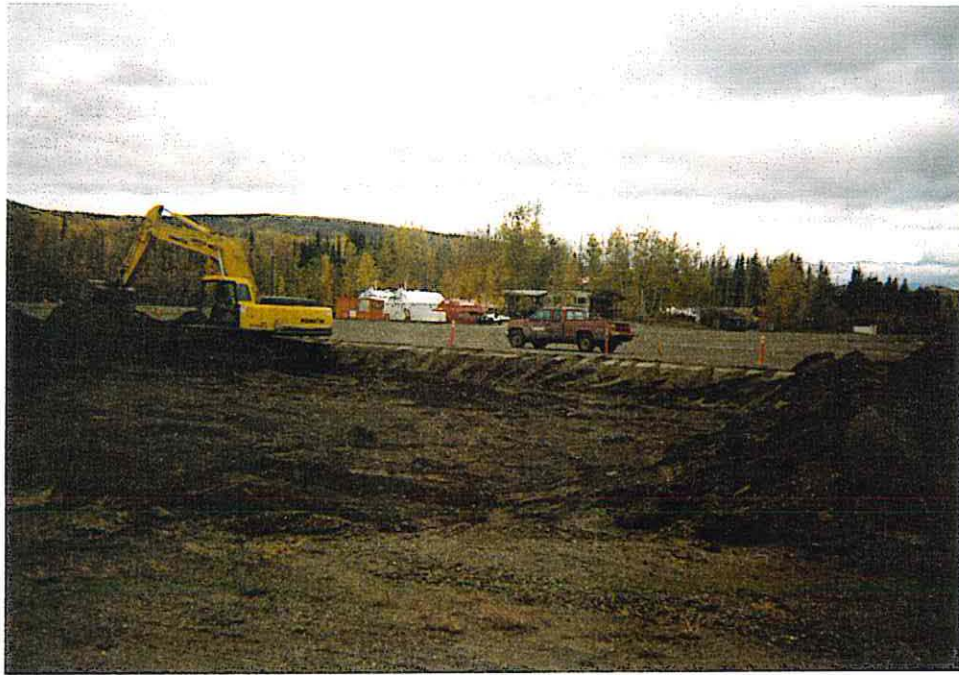
PHOTO # 14 – Repair Area 3-1 – Excavation Base
