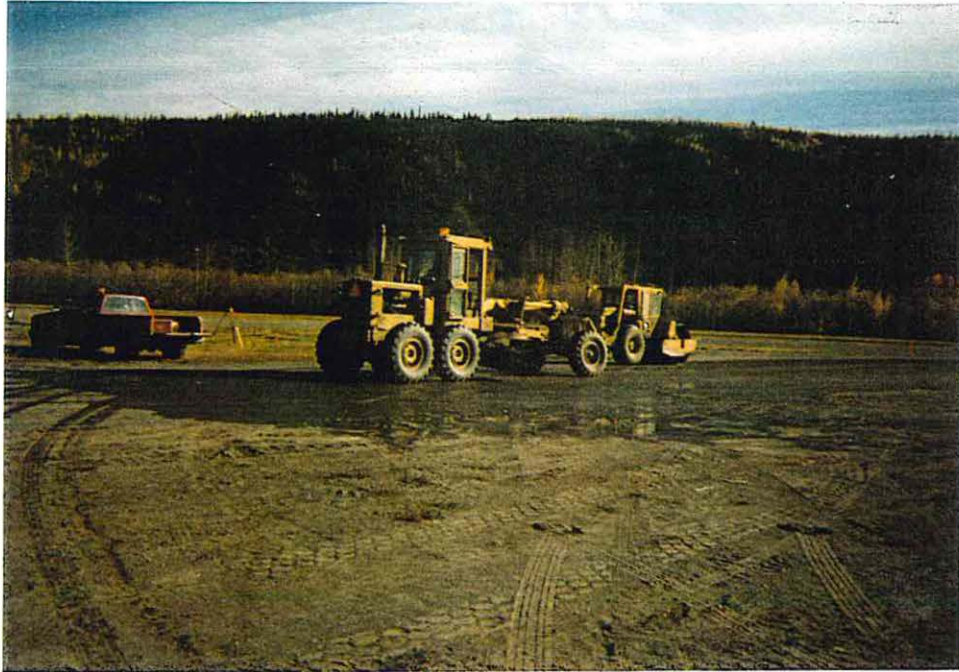
PHOTO # 8 – Repair Area 1 – Final Grading and Compacting
