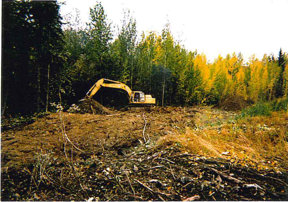
PHOTO # 1 – New Vehicle Parking Area – Clearing and Grubbing Operations
