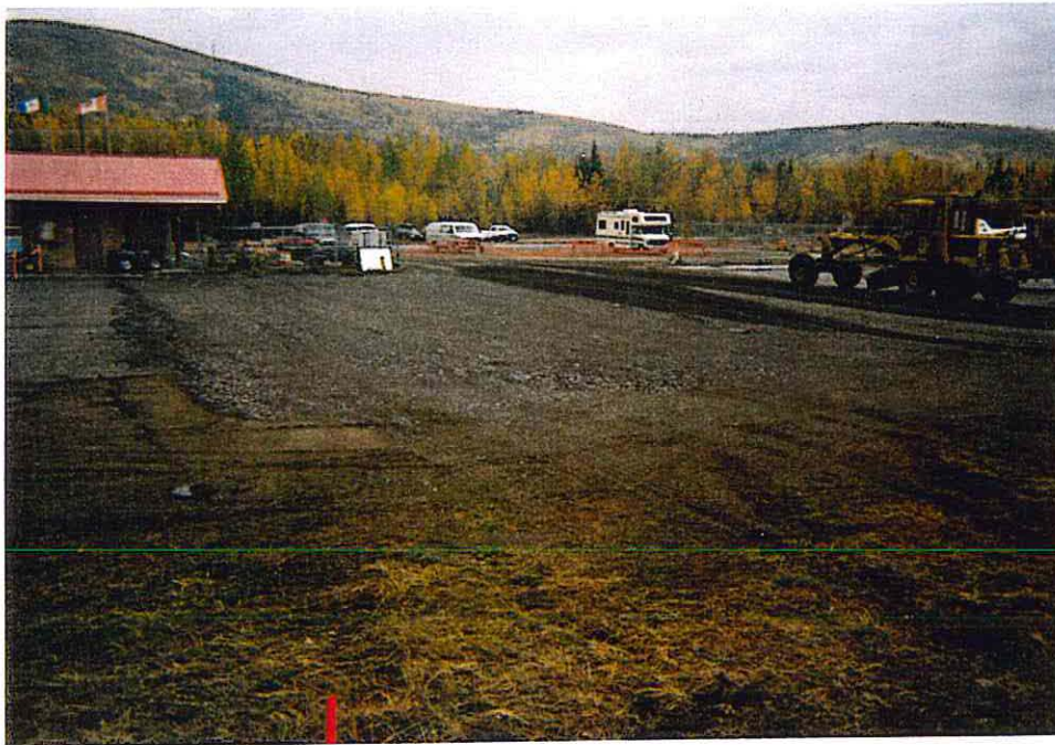
PHOTO # 13 – Repair Area 2 – Granular A Grading and Compaction
