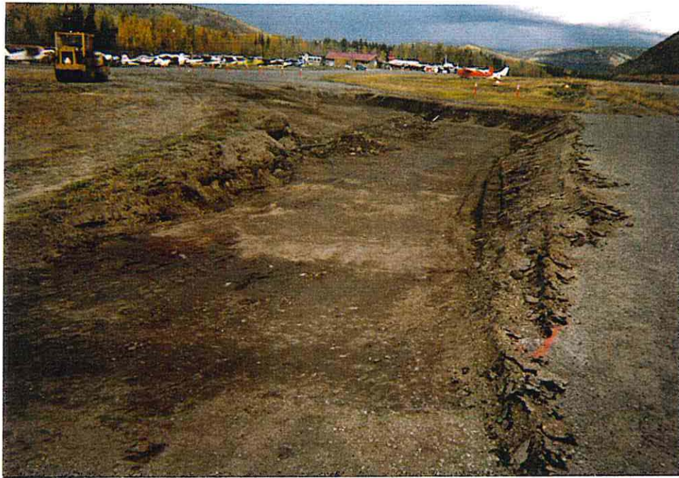
PHOTO # 5 – Repair Area 1 – Excavation Base Note location of VASES cable
