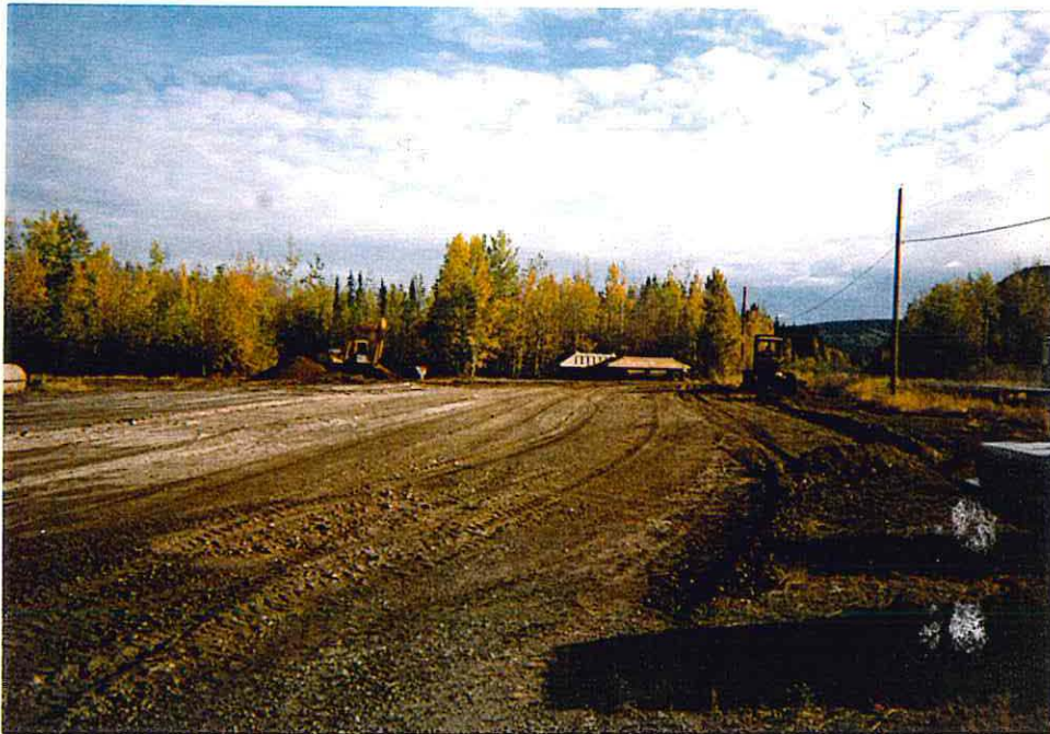
PHOTO # 2 – Existing Vehicle Parking Area – Grading Operations
