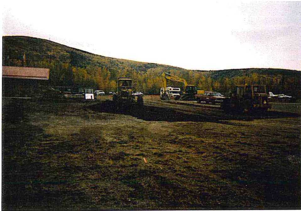
PHOTO # 12 – Repair Area 2 – Granular E Backfill Operations
