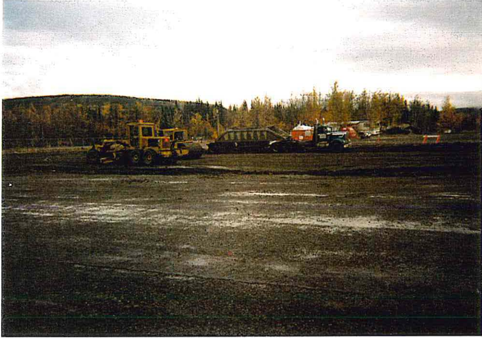
PHOTO # 15 – Repair Area 3-2 – Granular E Backfill Operations
