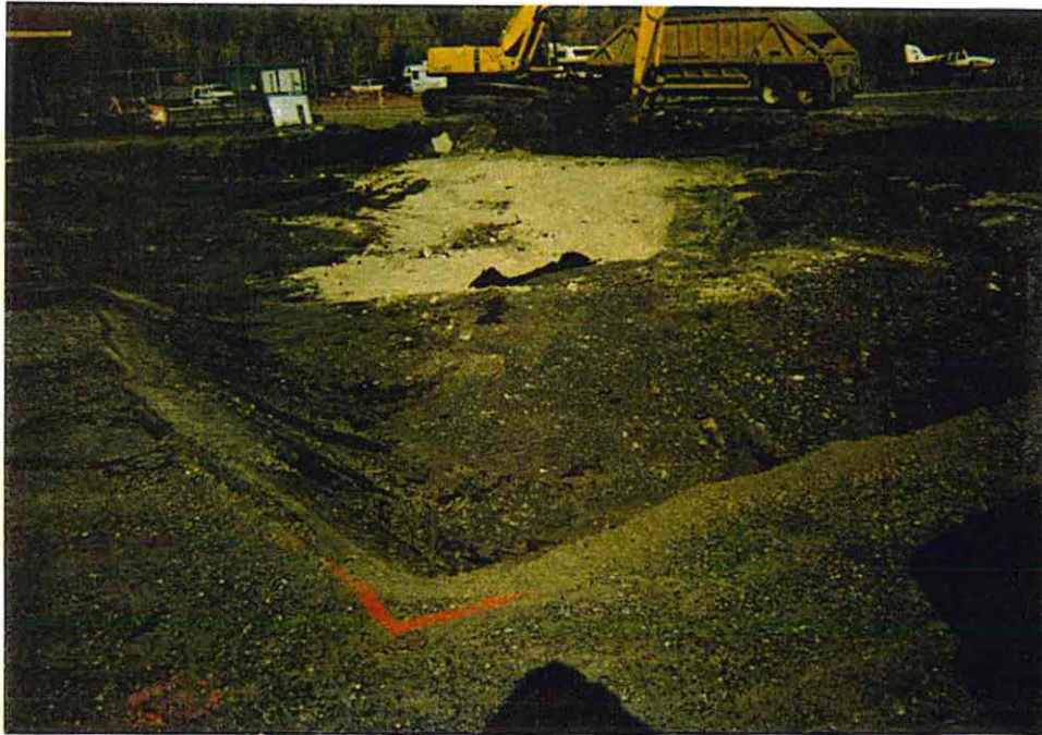
PHOTO # 10 – Repair Area 2 – Excavation Base
