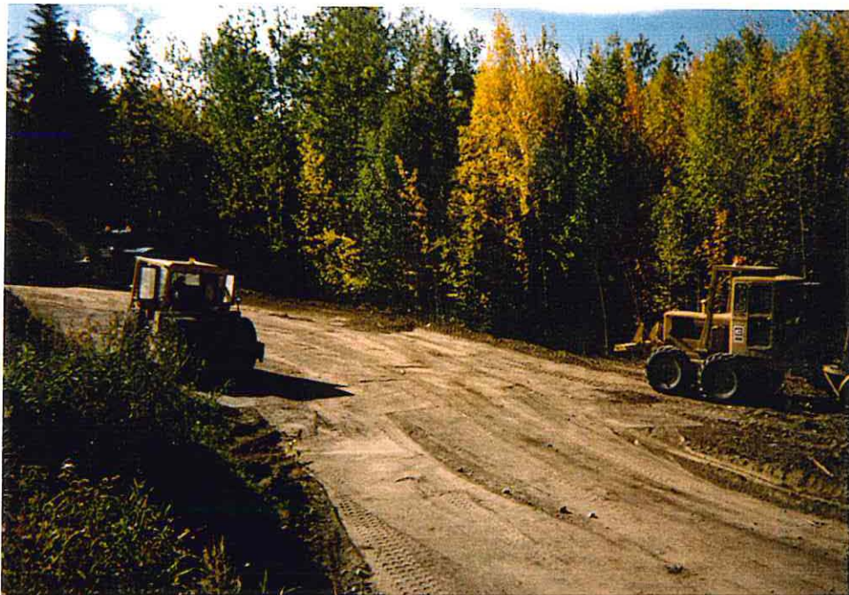
PHOTO # 3 – New Vehicle Parking Area – Construction of Subgrade (Southwest corner)
