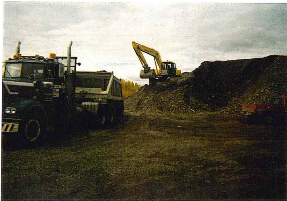
PHOTO # 11 – km 688.7 – Loading of Granular E material from existing stockpile.
