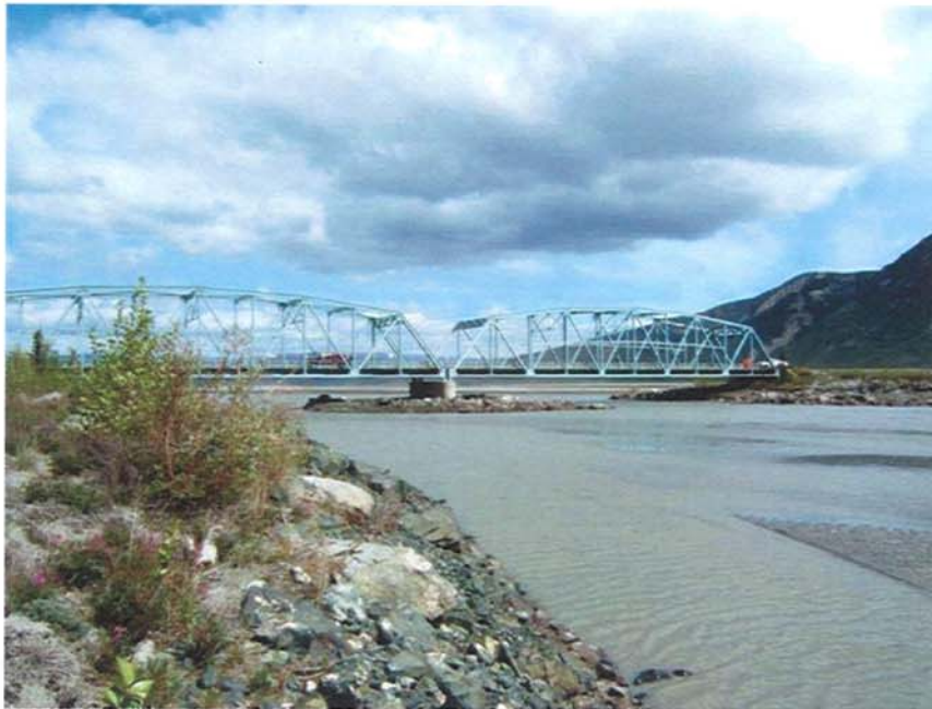
Floodplain of Slims River adjacent to the existing Bridge – Looking West
