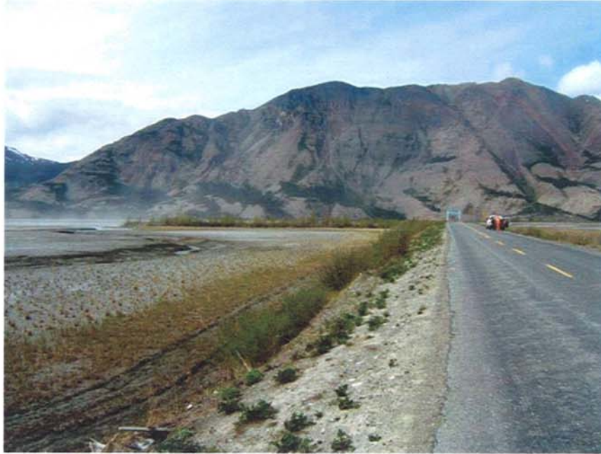
Photograph of Slims River Bridge – Looking North
