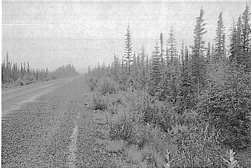
Figure 11: Large, low terrace surface that will be underlain by sand and gravel.
