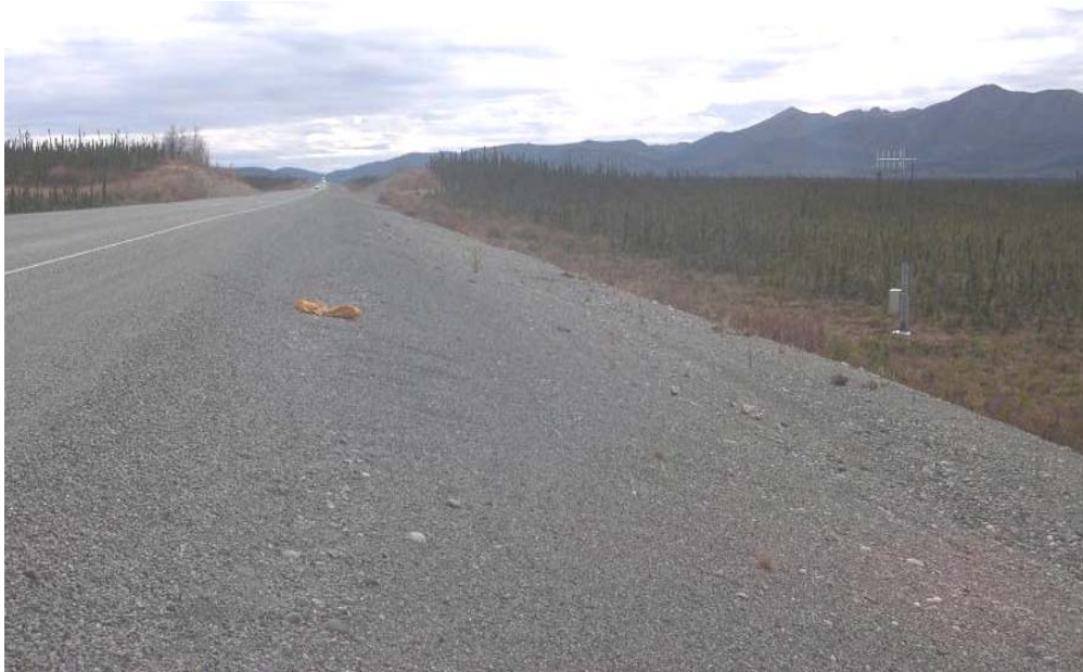
Figure 3-1: Temperature monitoring station on the Alaska Highway near Beaver Creek
