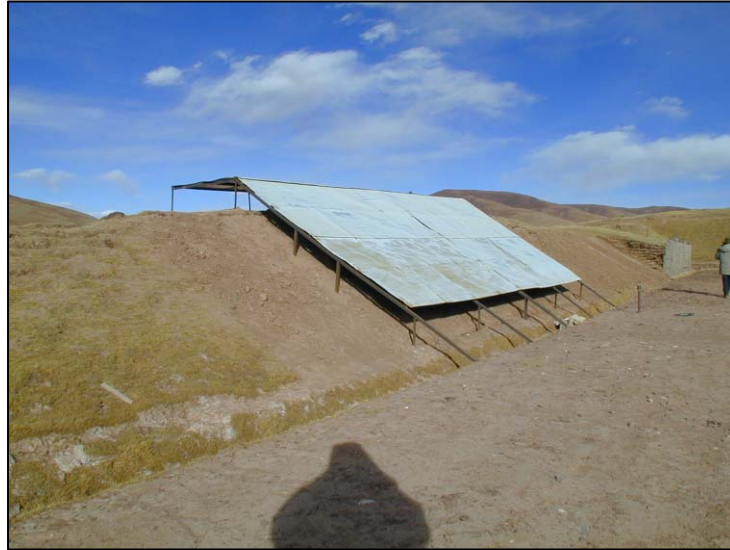
Figure 2-11: Sunsheds, Qinghai-Tibet Roadway, Tibetain Plateau (Courtesy of Professor Ma, Lanzhou, China)
