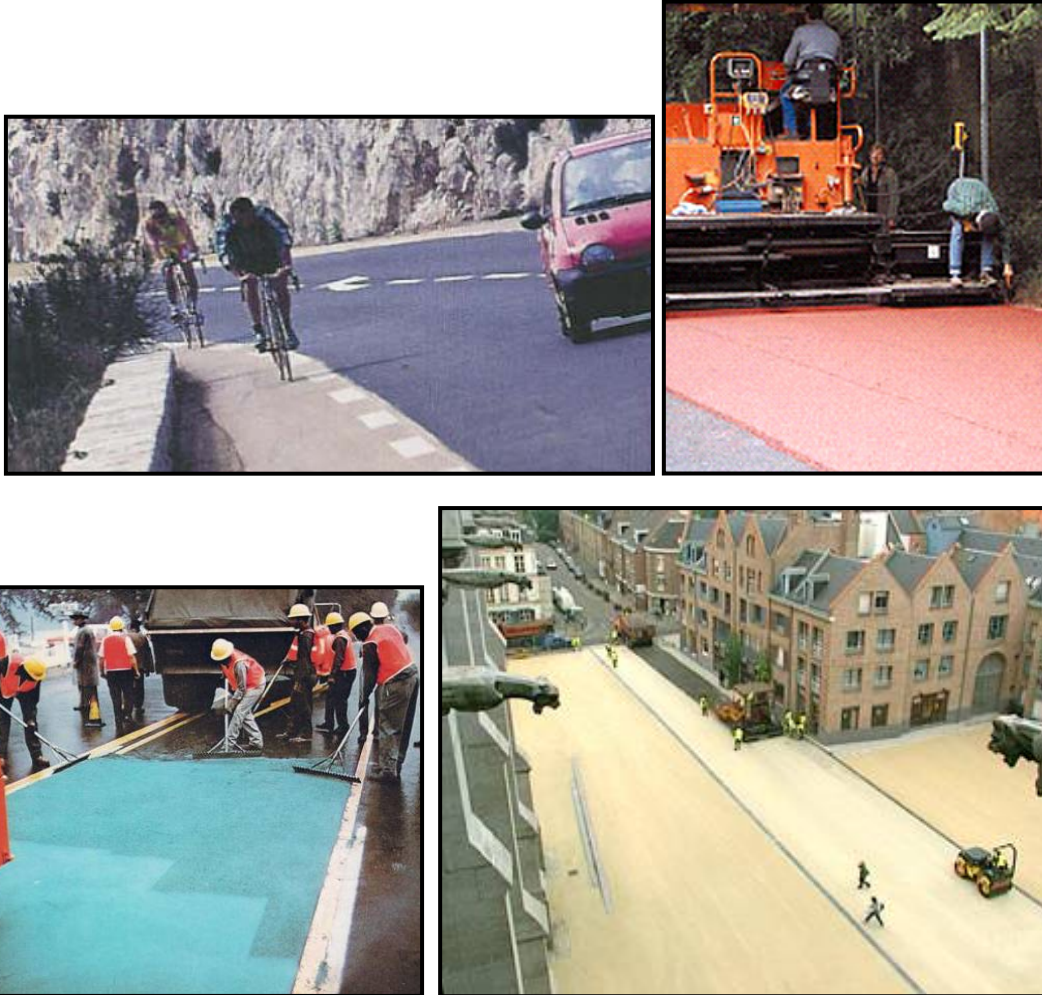
Figure 4-4: Coloured asphalt products used in Europe (Mexphalte C, patented by Shell)
