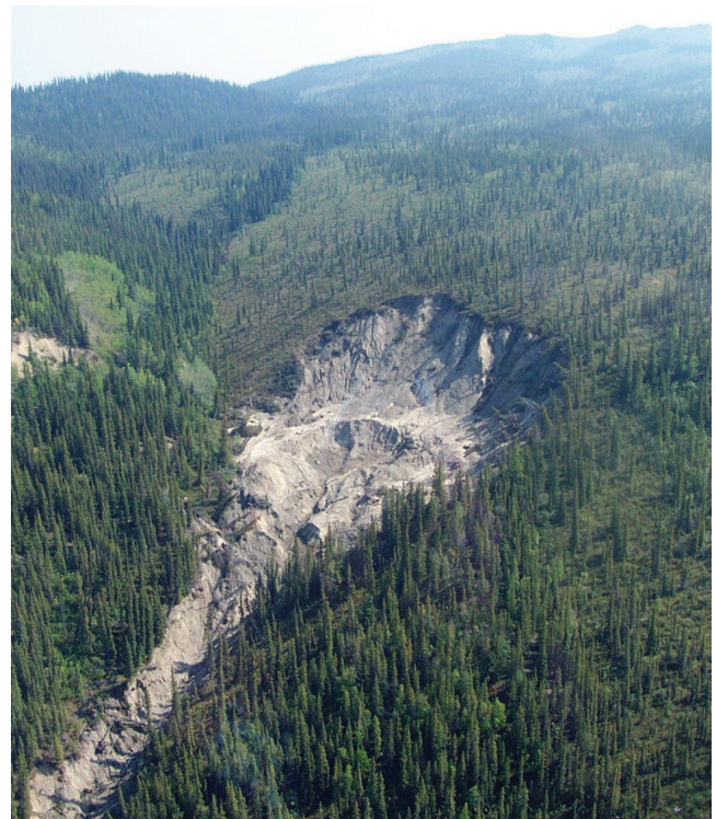
Figure 1. Aerial view of landslide source zone showing debris torrent channel exiting at lower left corner. Maximum height of the headwall is 31 m and the bowl is approximately 160 m wide.
