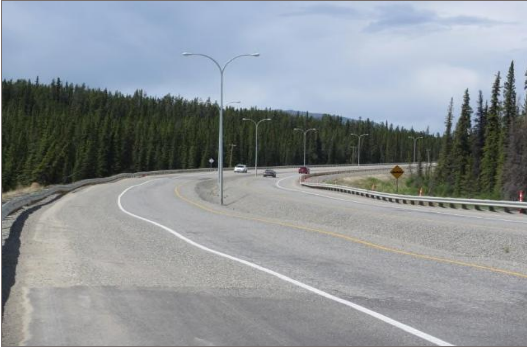
Photo 1: Hamilton Boulevard, aspect NW, June 11, 2013
