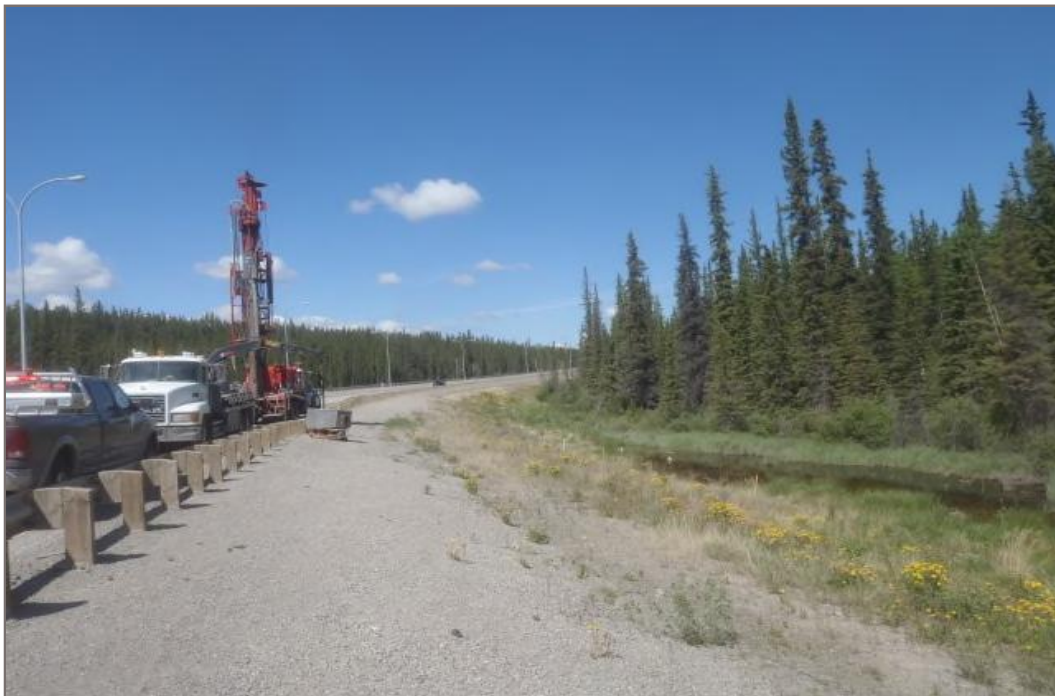
Photo 8: BH03 Setup, aspect NW
