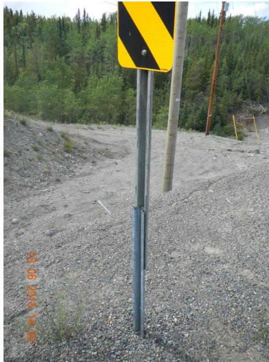
Picture 3-11 Typical sign post installation, long anchor and no breakaway.
