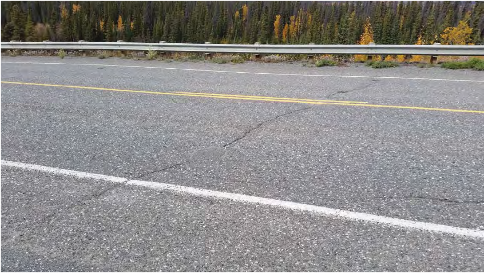
Marshal Creek Site Photo 3
