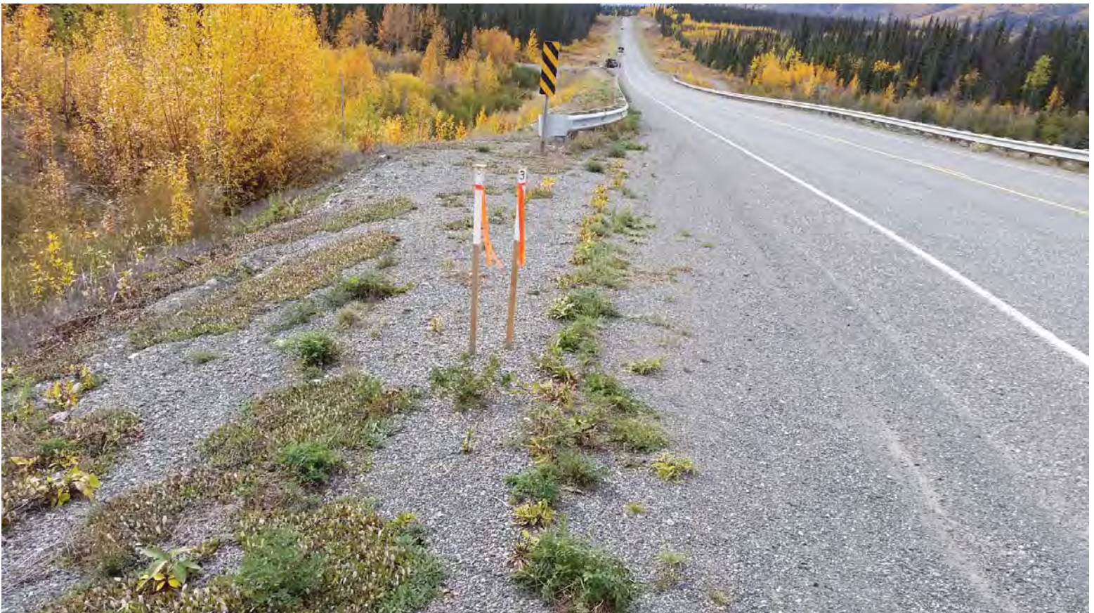
Marshal Creek Site Photo 2
