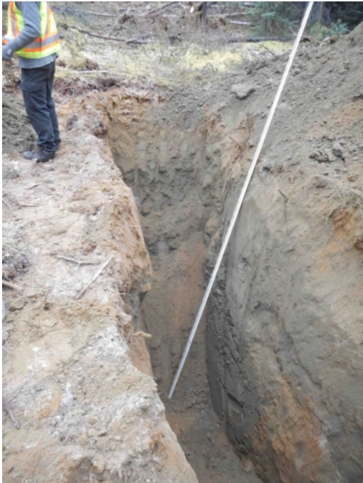
Figure 869-5330.4 Photo of Test Pit 5330
