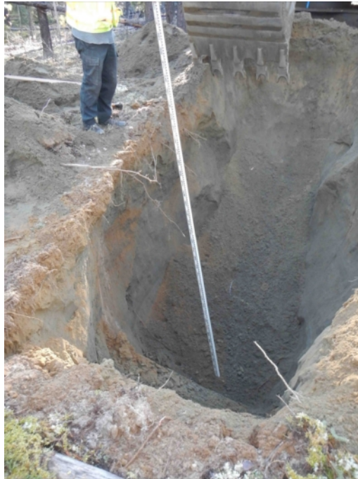
Figure 869-5328.4 Photo of Test Pit 5328
