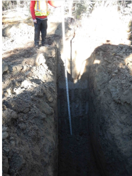
Figure 869-5322.5 Photo of Test Pit 5322
