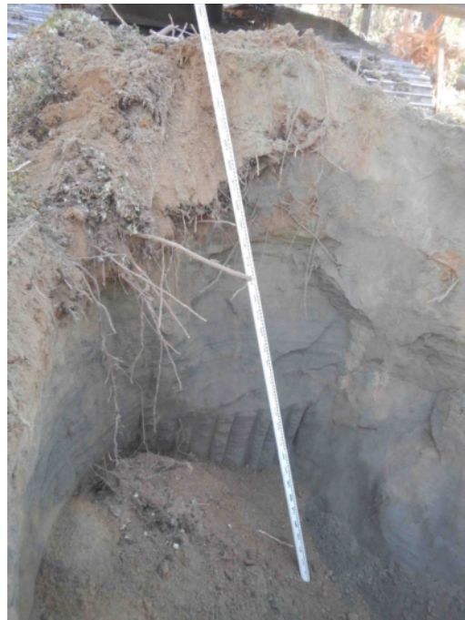
Figure 869-5327.4 Photo of Test Pit 5327
