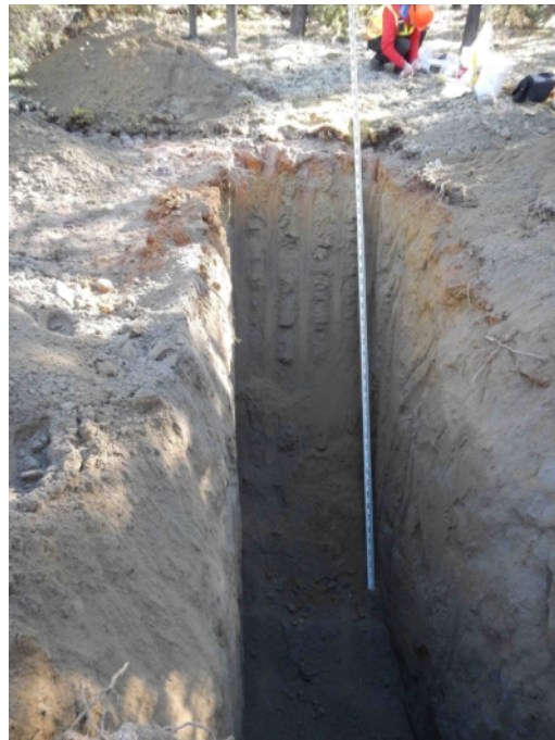
Figure 869-5323.4 Photo of Test Pit 5323
