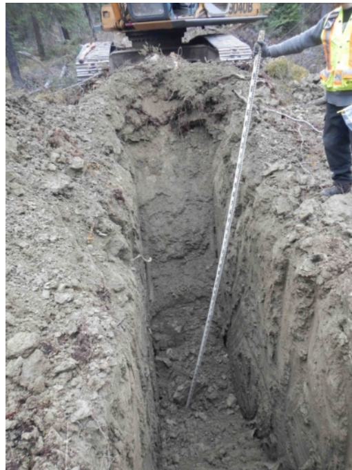
Figure 869-5333.4 Photo of Test Pit 5333
