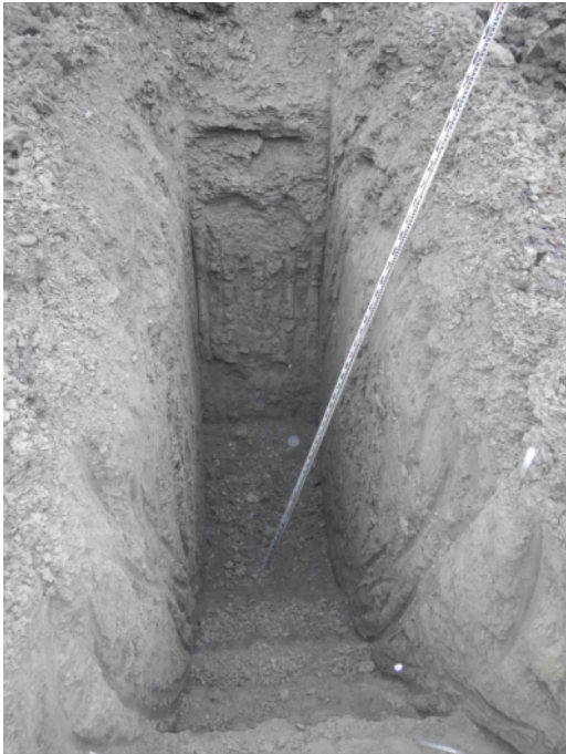
Figure 871-5353.4 Photo of Test Pit 5353
