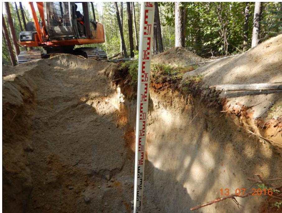
Figure 890-5658.2 Photo of test pit 890-5658
