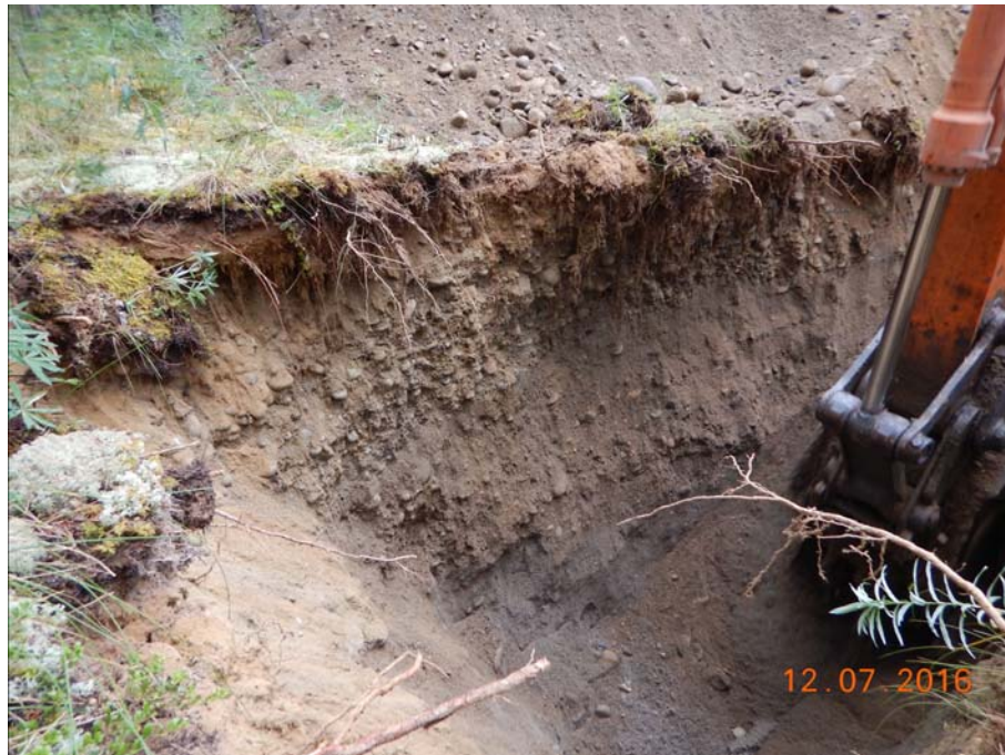
Figure 890-5660.2 Photo of test pit 890-5660
