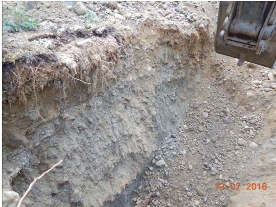
Figure 890-5670.2 Photo of test pit 890-5670
