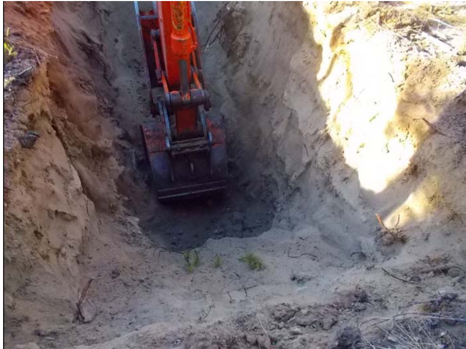
Figure 901-6585.1 Photo of test pit 901-6585
