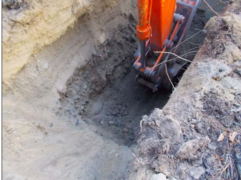
Figure 901-6580.1 Photo of test pit 901-6580
