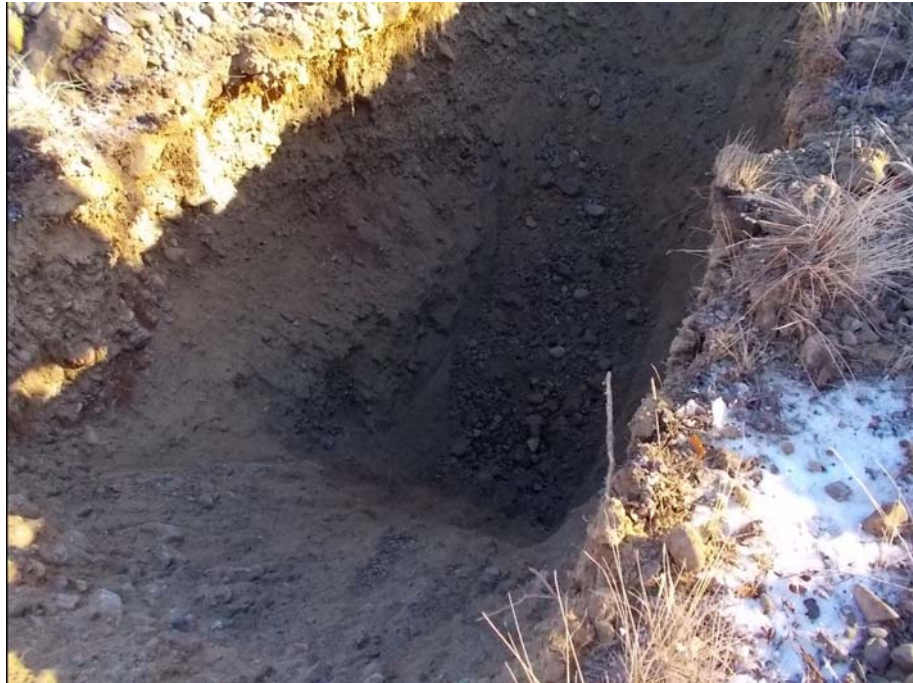
Figure 901-6583.1 Photo of test pit 901-6583
