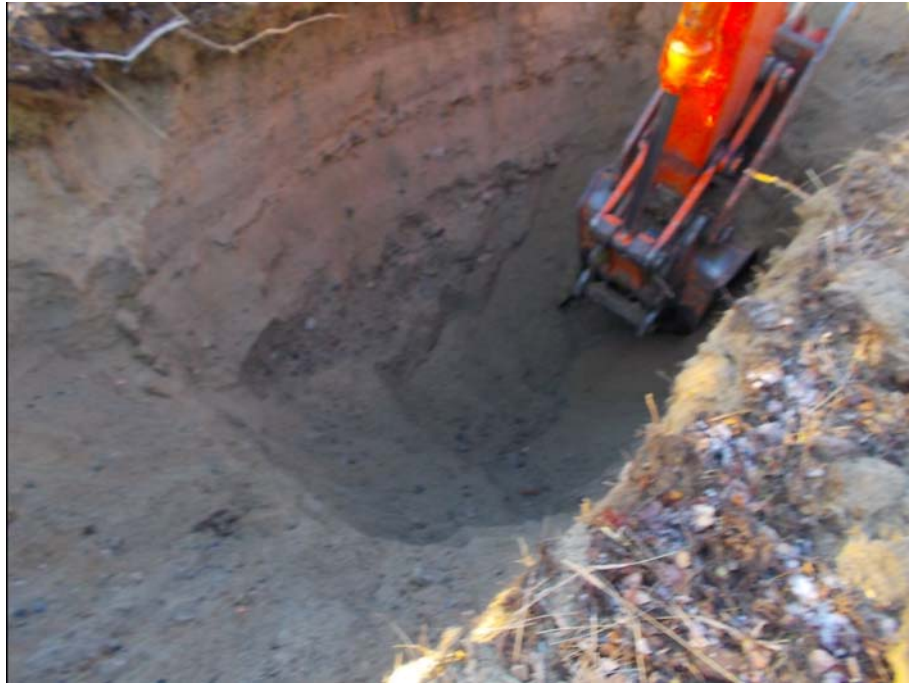
Figure 901-6587.1 Photo of test pit 901-6587
