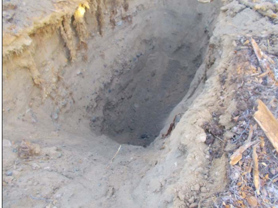
Figure 901-6581.1 Photo of test pit 901-6581
