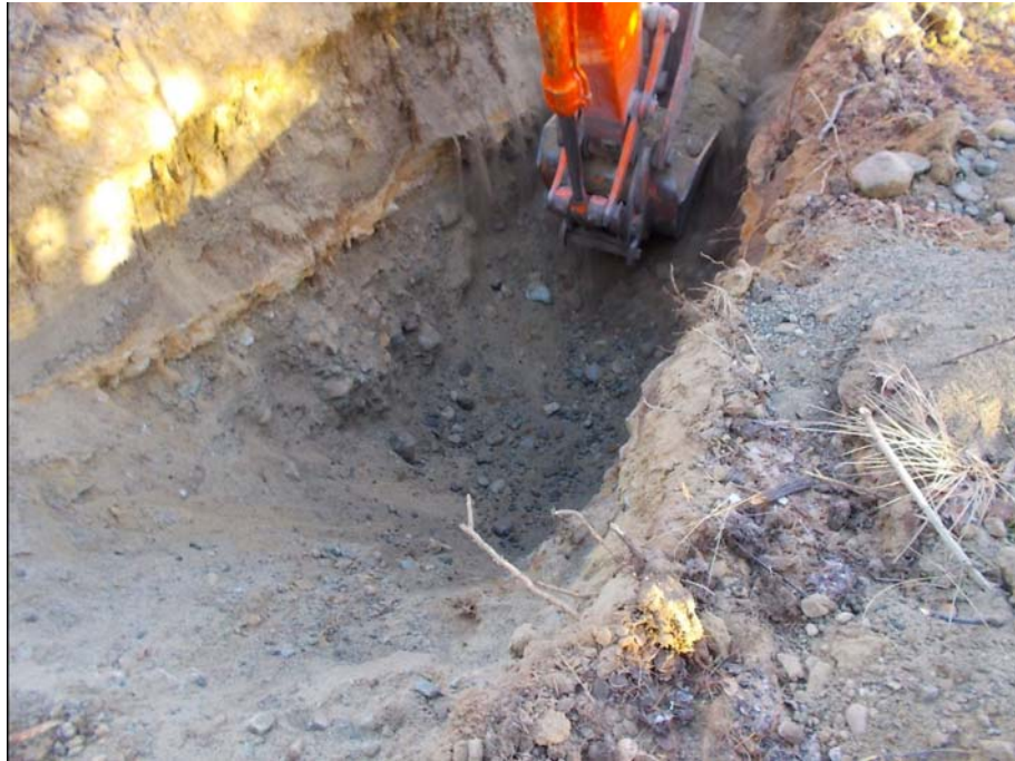
Figure 901-6582.1 Photo of test pit 901-6582
