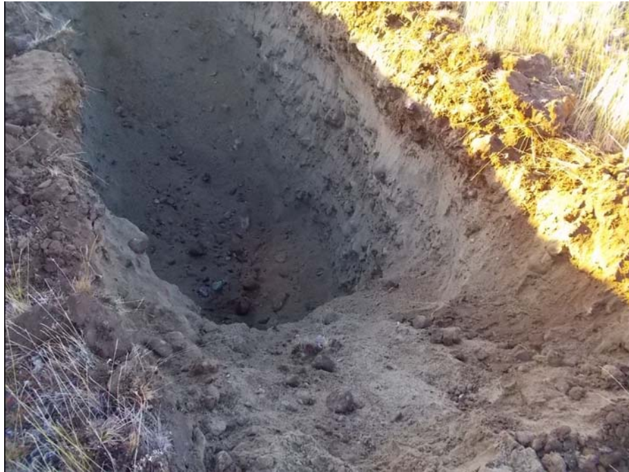
Figure 901-6590.1 Photo of test pit 901-6590
