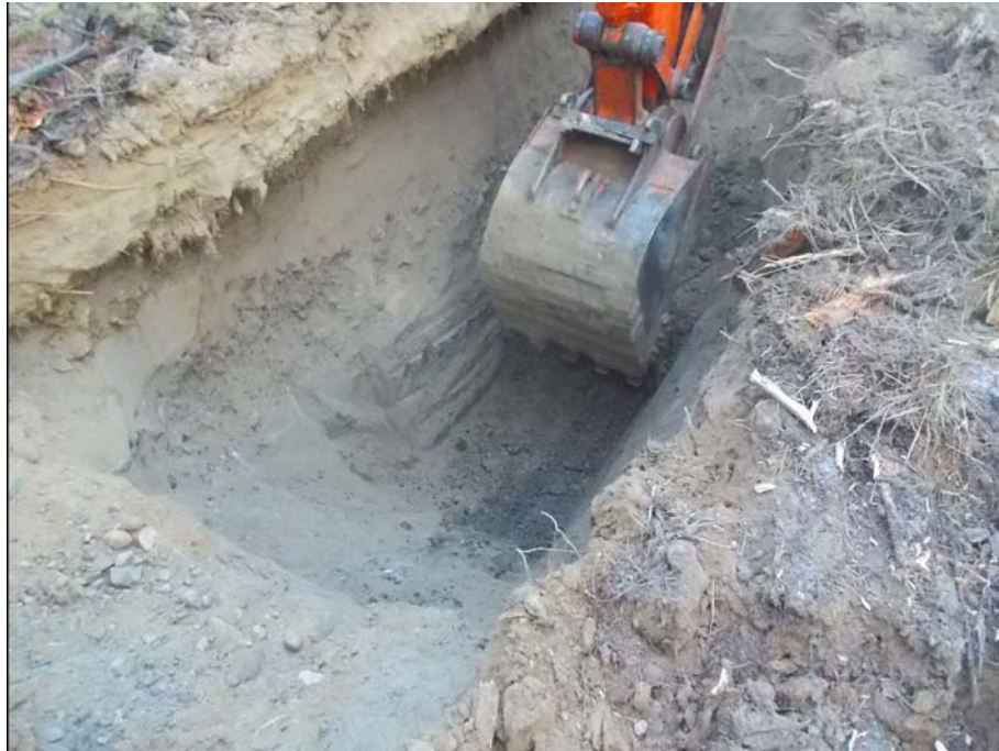
Figure 901-6579.1 Photo of test pit 901-6579
