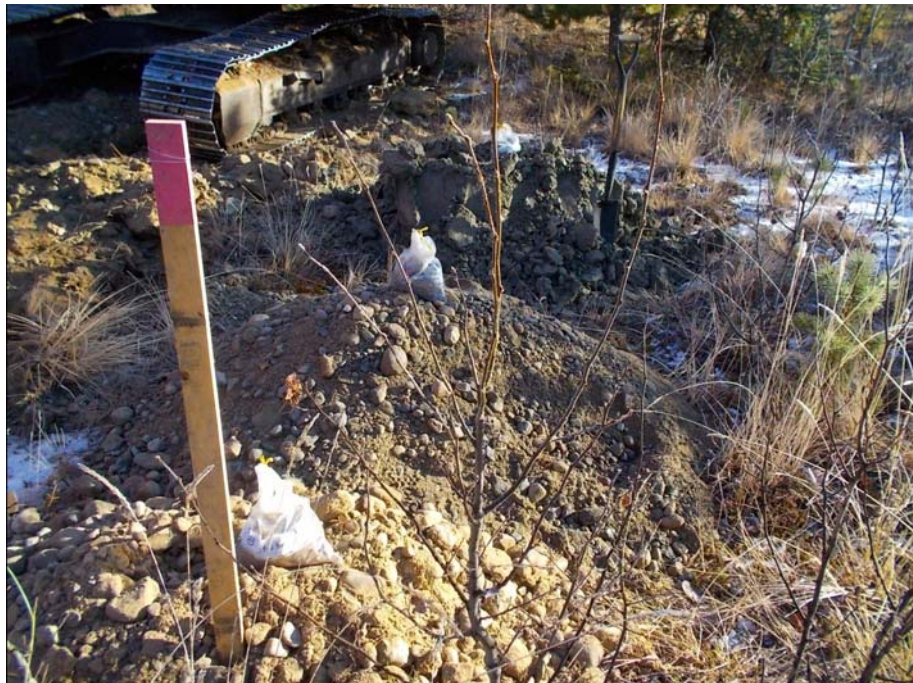
Figure 901-6583.2 Photo of sample piles from test pit 901-6583
