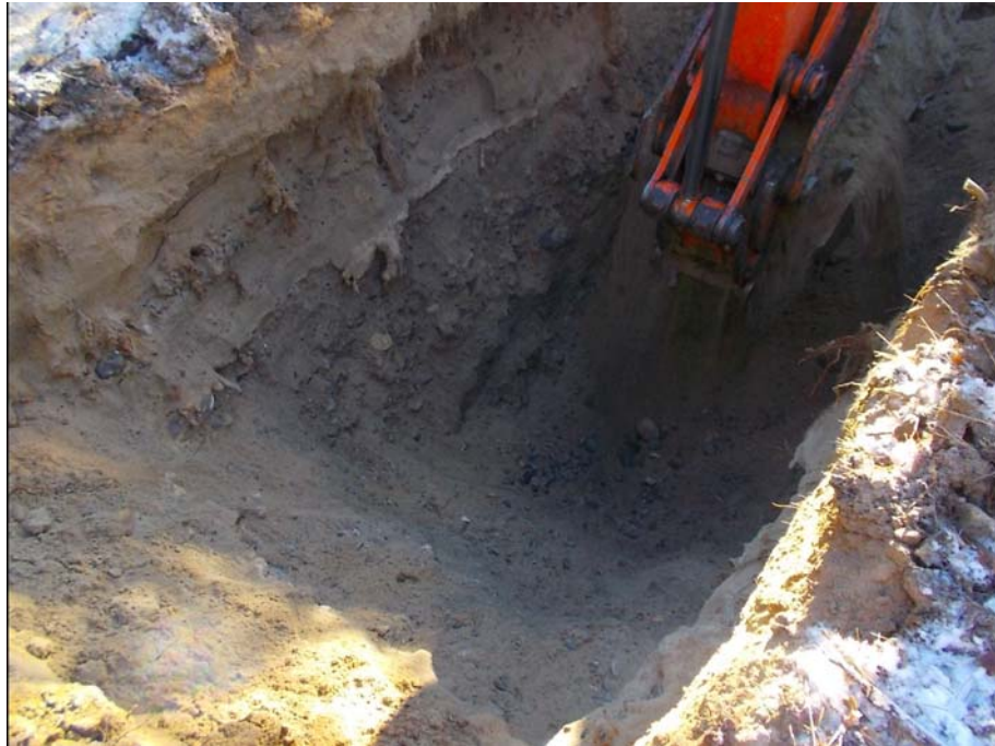
Figure 901-6586.1 Photo of test pit 901-6586
